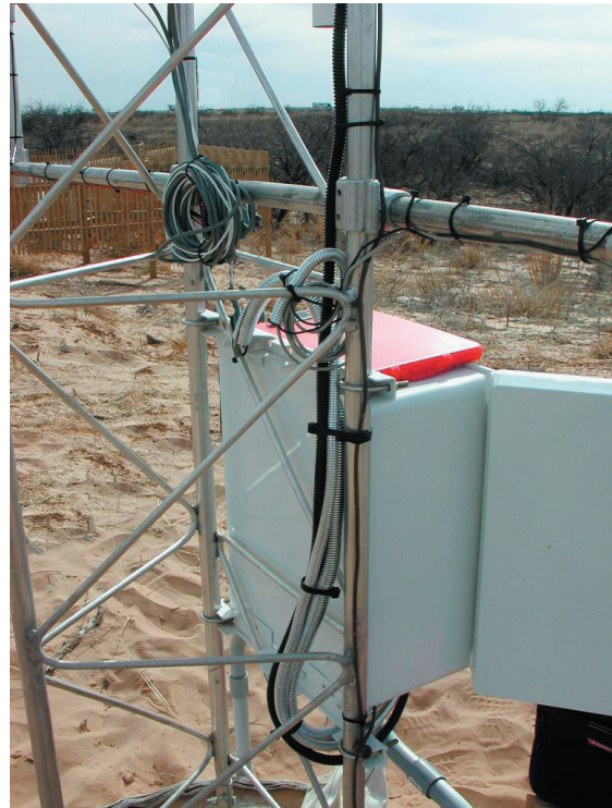
Figure 3: Completed installation of the protection of the cabling
