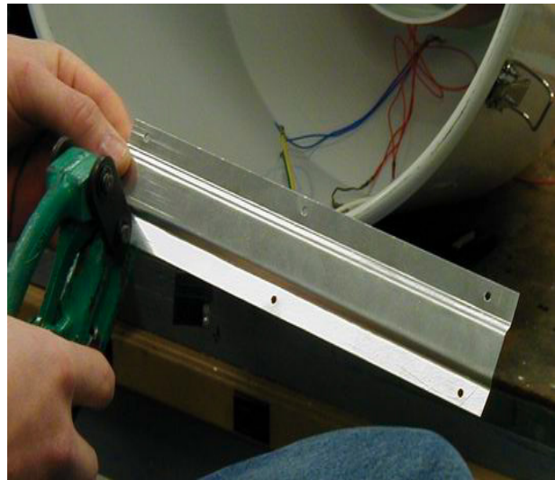
Figure 8: The metal protective wire cover is prepared for installing.
