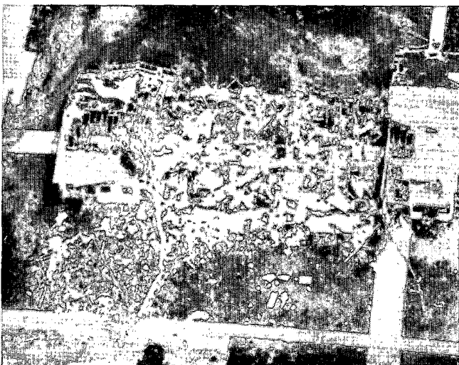
Left: Aerial photo of a tie-beam (see map) blown off toward the west. Fujita photo 1245 EDT 9/14/92. Right: Ground view of the tie-beam reinforced with one-inch steel rods. Fujita photo 1649 EDT 9/15/92.
