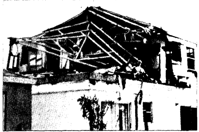
Above(left): This aerial view depicts the uneven damage pattern found in various wood structures in the Lakes By the Bay residential development. Above(right): A close-up view of a home in the development. The gable end of the roof failed during the storm. This was a frequent problem in homes of mixed wood and concrete block construction. (Photo courtesy: NHC)
