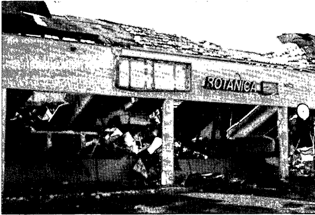
Above(left): Front view of the east (windward) face of a strip shopping center on the north side of Quail Roost Drive, near the Florida Turnpike. Winds flowing in through the broken plate glass windows, pushed the walls outward a sufficient distance to allow the pre-cast concrete roof to fall into the store. Above(right): View of the rubble inside a "Food Stop" convenience store, at the same shopping center. (Photo courtesy: Roger Edwards)
