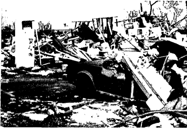
Above(left): Naranja Lakes homes were primarily concrete block and stucco (or CBS) construction. The force of Andrew's wind was strong enough to lift concrete tie beams and propel them into nearby structures. Above(right): This home in Naranja Lakes shows inadequate tie beam construction. Note that there were no vertical ties to the foundation. Many homes in Naranja Lakes lacked any vertical tie columns. (Photo courtesy: NHC)
