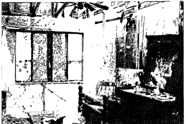
Above(left): The frame is all that remains of this mobile home. This demonstrates the high risk to residents who must ride out severe wind storms in such a structure. Above(right): A damaged home in the Saga Bay development clearly shows the damage inflicted by high wind and heavy rain. Insulation is splattered across the bedroom walls. (Photo courtesy: NHC)
