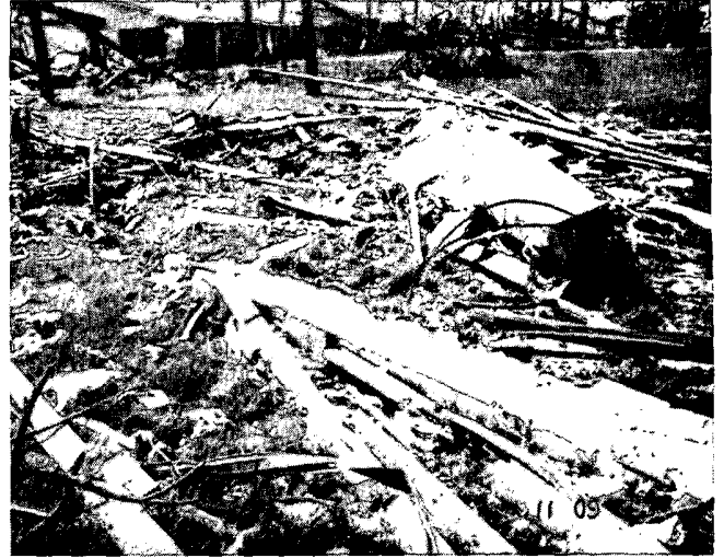
Left: Tie-beams at Pine Woods Villa (see map) blown apart by a mini-swirl. Continental Aerial Survey photo taken on 8/27/92. Right: Ground view of the tie-beams. Fujita photo 1109 EDT 9/9/92.
