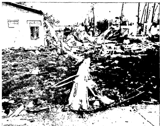
Left: Aerial photo of a tie-beam (see map) blown off toward the west. Fujita photo 1245 EDT 9/14/92. Right: Ground view of the tie-beam reinforced with one-inch steel rods. Fujita photo 1649 EDT 9/15/92.
