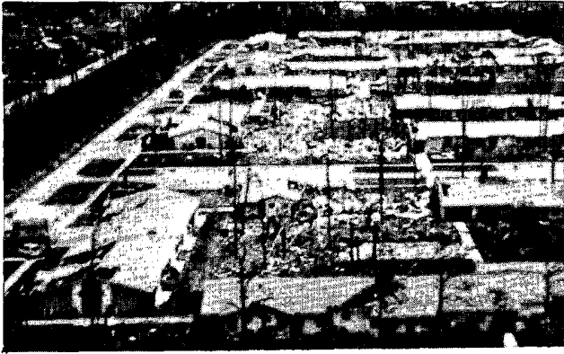
Above(left): This aerial view of a section of Pinewoods Villa, a development located in Whispering Pines, shows an uneven damage pattern. Also note the roof damage to the building located in the center foreground. This damage resulted from a tie beam that was torn from a home 300 feet away and then dropped through the roof of the structure. Above(right): A view of the tie beam from inside the structure. This type of tie beam typically weighs at least 1,000 pounds! (Photo courtesy: NHC)
