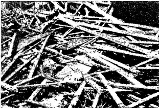
Above(left): Many roof trusses failed during the hurricane force winds. Above(right): These rustic shops were part of Gauley Square, a shopping area located north of Homestead. Both new and old buildings suffered significant damage. (Photo courtesy: NHC)
