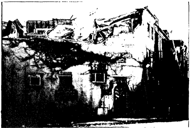
Above(left): Many roof trusses failed during the hurricane force winds. Above(right): These rustic shops were part of Gauley Square, a shopping area located north of Homestead. Both new and old buildings suffered significant damage. (Photo courtesy: NHC)
