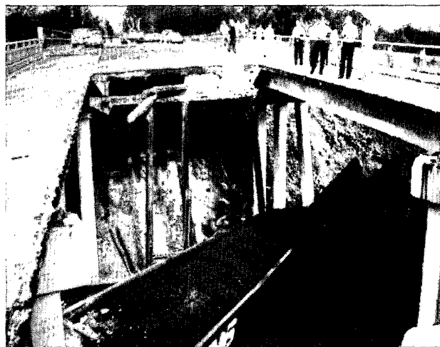
A 60-foot section of a railroad overpass (Highway 176) in St. Matthews, SC fell 30 feet when a freight train derailed and struck the overpass supports. Derailment was blamed on 24-hour rains of 12.30 inches and washed out tracks. Two vehicles plummeted off the overpass resulting in one death and one serious injury. Photo credit: Wes Tyler, S.C. State Climatology Office.
