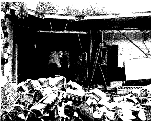
Remains of the Haile Street Grill in Camden, SC after being hit by the water released by the break in the Kendall Lake Dam. Photo courtesy: Chronicle-Independent, Camden, SC.
