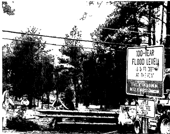
Repair crew working on a bridge on Haile Street after the failure of Kendall Lake Dam in Camden, SC. Photo courtesy: Chronicle-Independent, Camden, SC.
