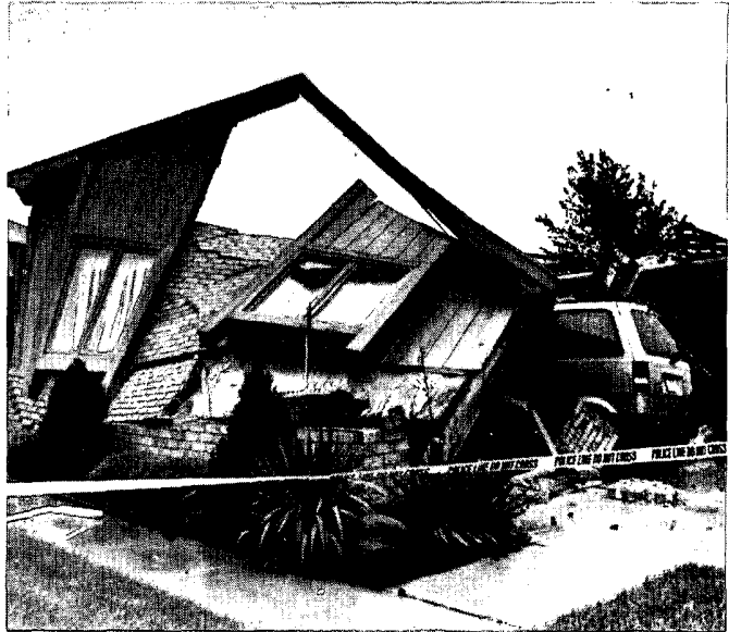
Tornado collapsed brick and frame wall of a residence in Novi. Note that the windows are unbroken. Photo courtesy: Novi (Michigan) News.
