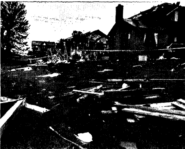
Severely damaged home in Novi after being hit by the F3 tornado. Debris, mostly from the home in center of photo, was scattered in a neighbor's backyard. Photo courtesy: Bryan Mitchell, Novi (Michigan) News.
