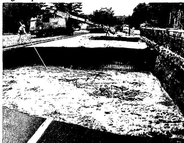
Washed out section of Highway 23 in Fond Du Lac. Richard Randall, District Bridge Safety Inspector, checks undermining of culvert footings. Reprinted with permission of the Duluth News-Tribune, Duluth, MN.
