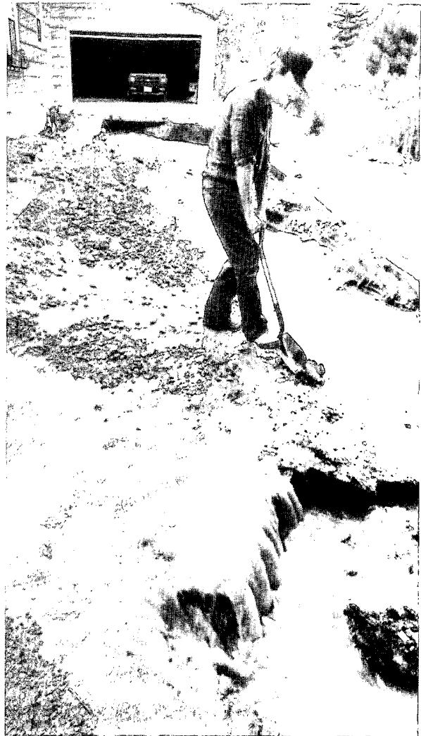
Driveway and garage foundation, owned by Mr. Ray Billings of Duluth, MN, suffered extensive flood/rain damage on September 5-6. Reprinted with permission of the Duluth News-Tribune, Duluth, MN.
