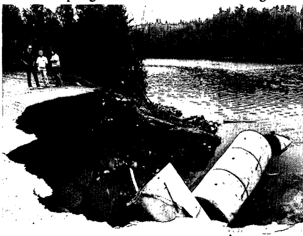
Engineers and a highway maintenance supervisor surveying flash flood damage to Highway 210 at Jay Cooke State Park. Reprinted with permission of the Duluth News-Tribune, Duluth, MN.
