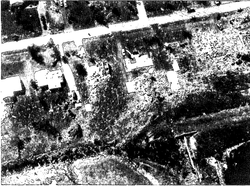
Left (top): Damage in the western section of Crest Hill. "Weaker" structures were generally blown off their foundations.
