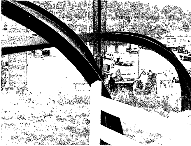
Left: This 75-foot-tall Waffle House sign at Harrison, Ohio was bent to the ground. The supports were 18 inches wide, made of 5/8-inch-thick steel, and buried in 12 feet of concrete. The sign was engineered to withstand 250 mph straight-line winds. Photo courtesy: Phillip Manuel, NWS Cincinnati.
