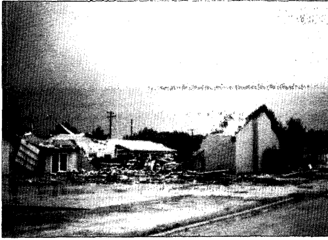
Left: Tornado damage to the Church of Christ in Spearman by the tornado shown on the preceding page. It was the fifth tornado of the day observed by the photographer and his crew. Photo courtesy and ©: Howard B. Bluestein; University of Oklahoma.
