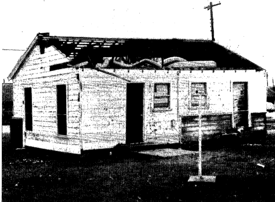
Photograph 1. The roof on this house was not anchored very well and was uplifted and displaced during peripheral winds in the Mesquite, Texas tornado on December 13, 1984. Wind velocities less than 100 m.p.h. can cause such residential damage.
