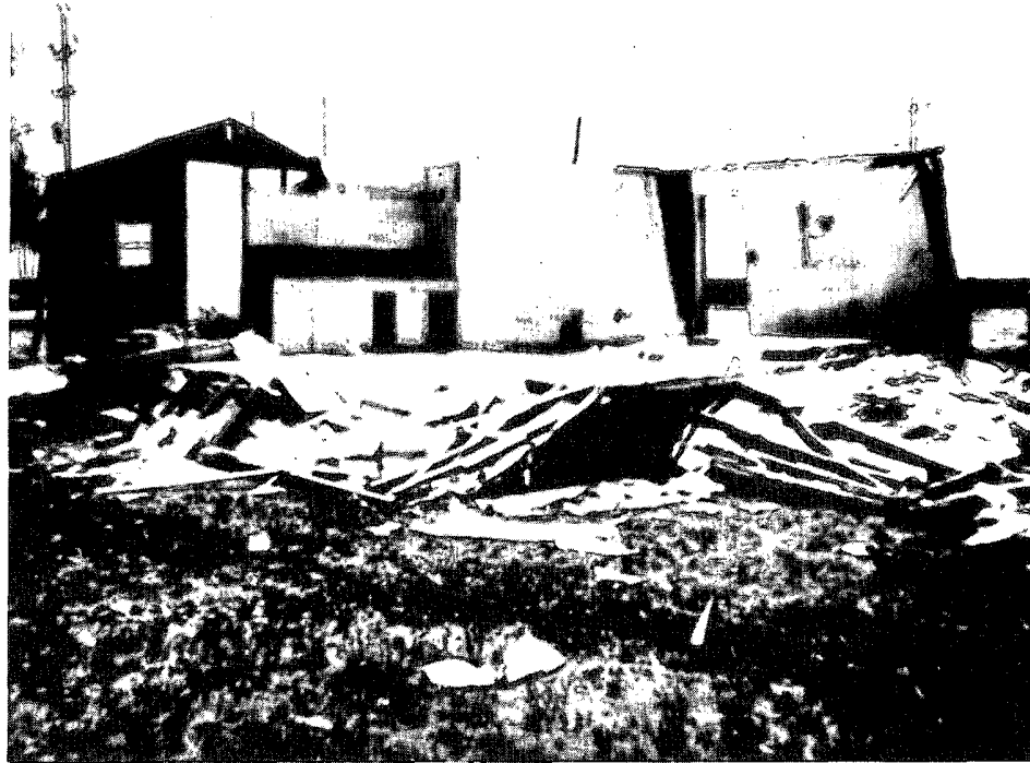
Photograph 8. At first glance, it may appear that this building exploded during this tornado. However, closer inspection reveals the back wall (at right) is leaning inward indicating this was the windward wall during the storm. Loss of the door and window allowed wind pressures to gain access to the building interior. Lack of roof/wall anchorage led to removal of the roof structure, and the remaining walls, no longer supported at the top, fell outward. Photograph courtesy of the Institute for Disaster Research at Texas Tech. University.
