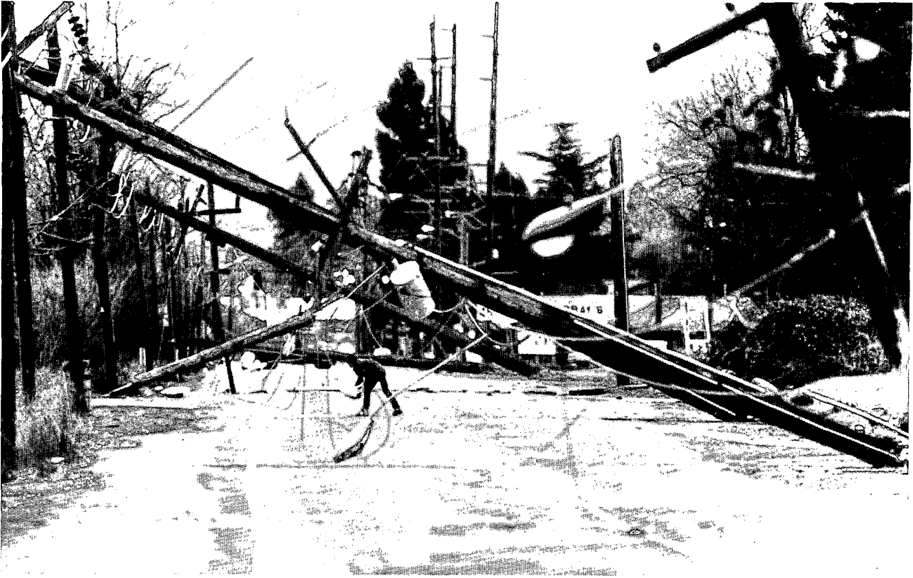
Wind damage in Portland, OR caused by January 9th storm. Photo by Kraig Scattarella, Oregonian Publishing Company, Portland, OR. Supplied by Tom Ainsworth, WSFO Portland, OR.
