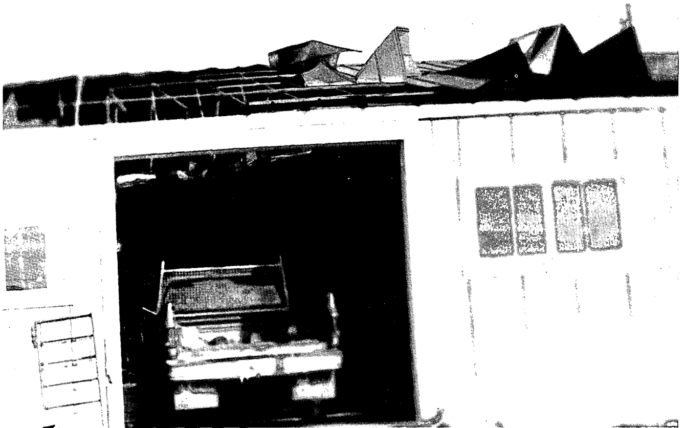
Wind damage in Buffalo, Wyoming on January 10th. Unofficial reports of wind gusts exceeding 120 mph. Photo by Carol Herman, Buffalo Bulletin. Supplied by Edward Berry, WSO Cheyenne.
