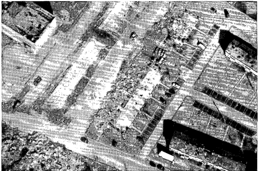
An overhead view of apartment building foundations immediately south of the Westbury Mall. Ground investigation of the site revealed that the two-story structures had no perceivable bolting system to their foundations, perhaps explaining in part the apparent ease with which the tornado swept these sizable structures away. Here, bulldozed (left) and unbulldozed (center) foundations can be compared.
