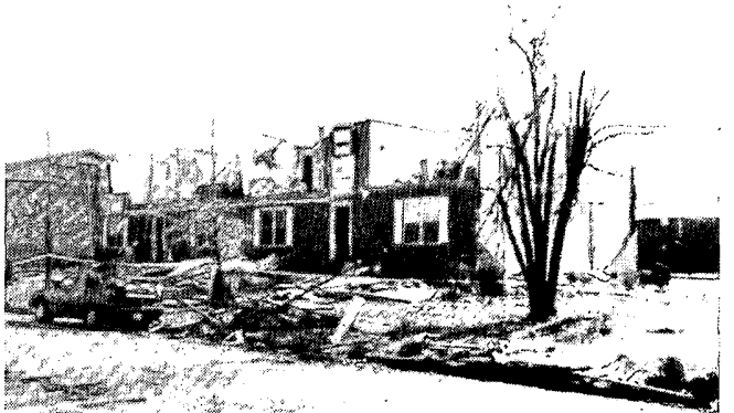
Only a small bit of the second level on this two-story apartment building was left by the tornado, the rest of the level having been scattered as debris to the structure's northeast (foreground).
