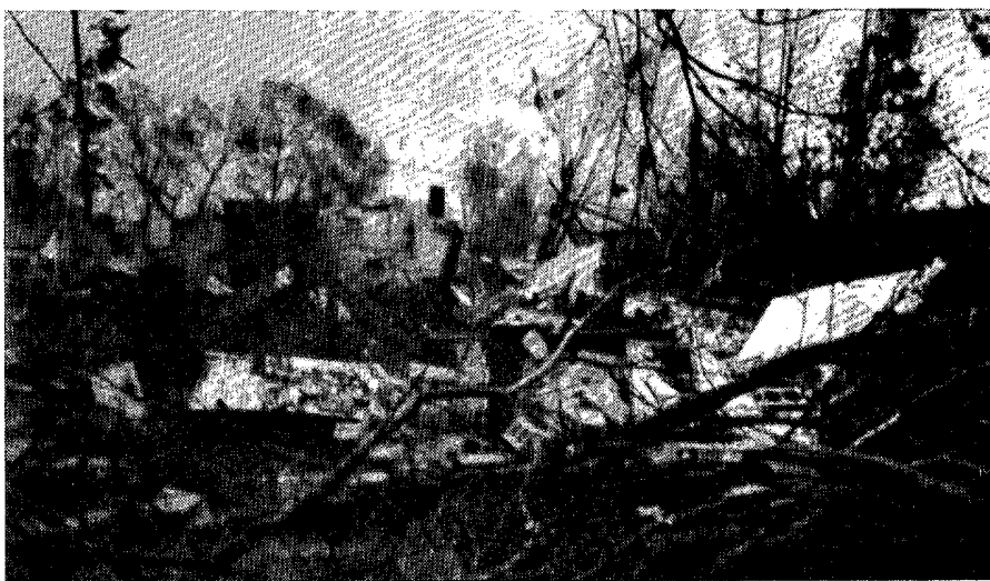
The rubble of a destroyed home in Alorton where the downburst winds were estimated at 100 mph.
