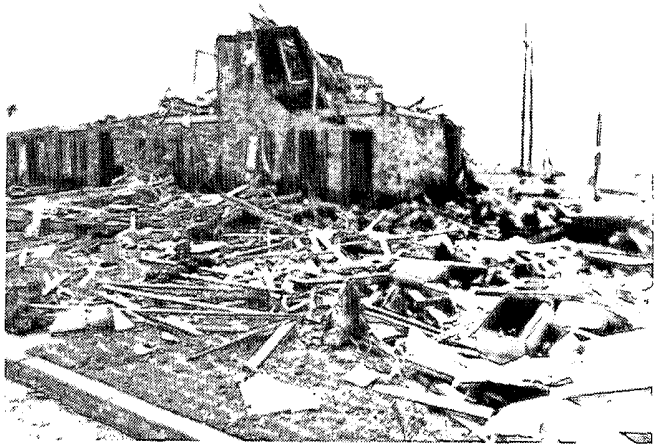
Only a small bit of the second level on this two-story apartment building was left by the tornado, the rest of the level having been scattered as debris to the structure's northeast (foreground).
