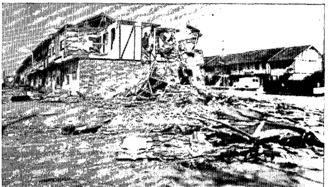
Damage to other two-story apartment buildings at the southern edge of the tornado's path, about one block south of the Westbury Mall.
