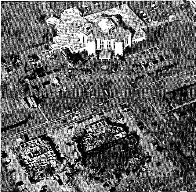
LEFT: Unroofed office buildings and nearby Crestwood Hospital (top of photo), all located on the north side of Airport Road, were structures that experienced the tornado's lesser winds at a given moment, being that they were caught in the left side of the vortex where its counterclockwise rotating winds opposed its direction of motion. The hospital received only minor damage, while its close proximity to the heavy damage area proved to be an asset in speeding the injured to the closest available medical attention. RIGHT: One of the office buildings of the Crestwood Professional Center is seen in two ground-level views from Airport Road. One vehicle had been tossed into the front of the building by the tornado.
