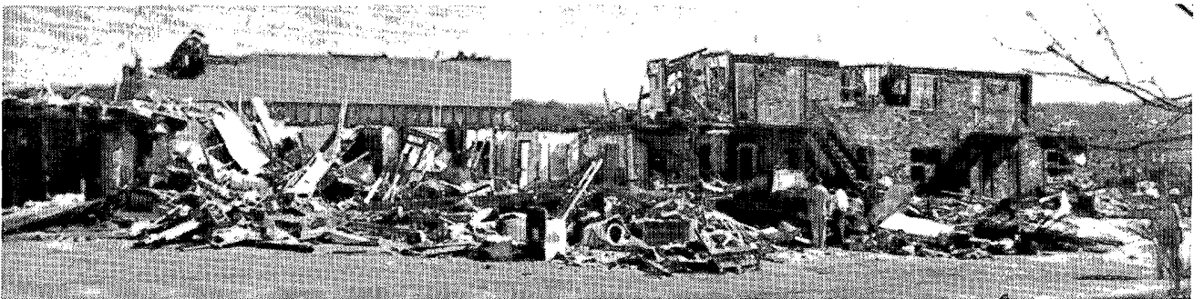
This apartment building immediately east of Memorial Parkway and south of Airport Road, lost its entire roof and half of its second floor, and even some of its first floor walls had been demolished. The view, of the building's rear, is toward the east.
