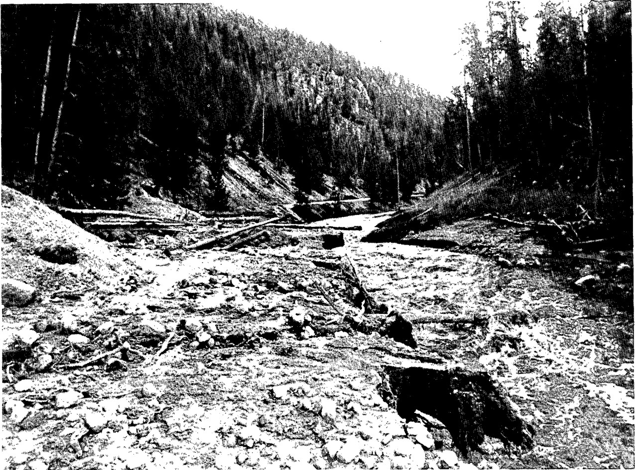
The portion of the roadway near Gibbon Falls that was covered by the worst of the mud slides.
