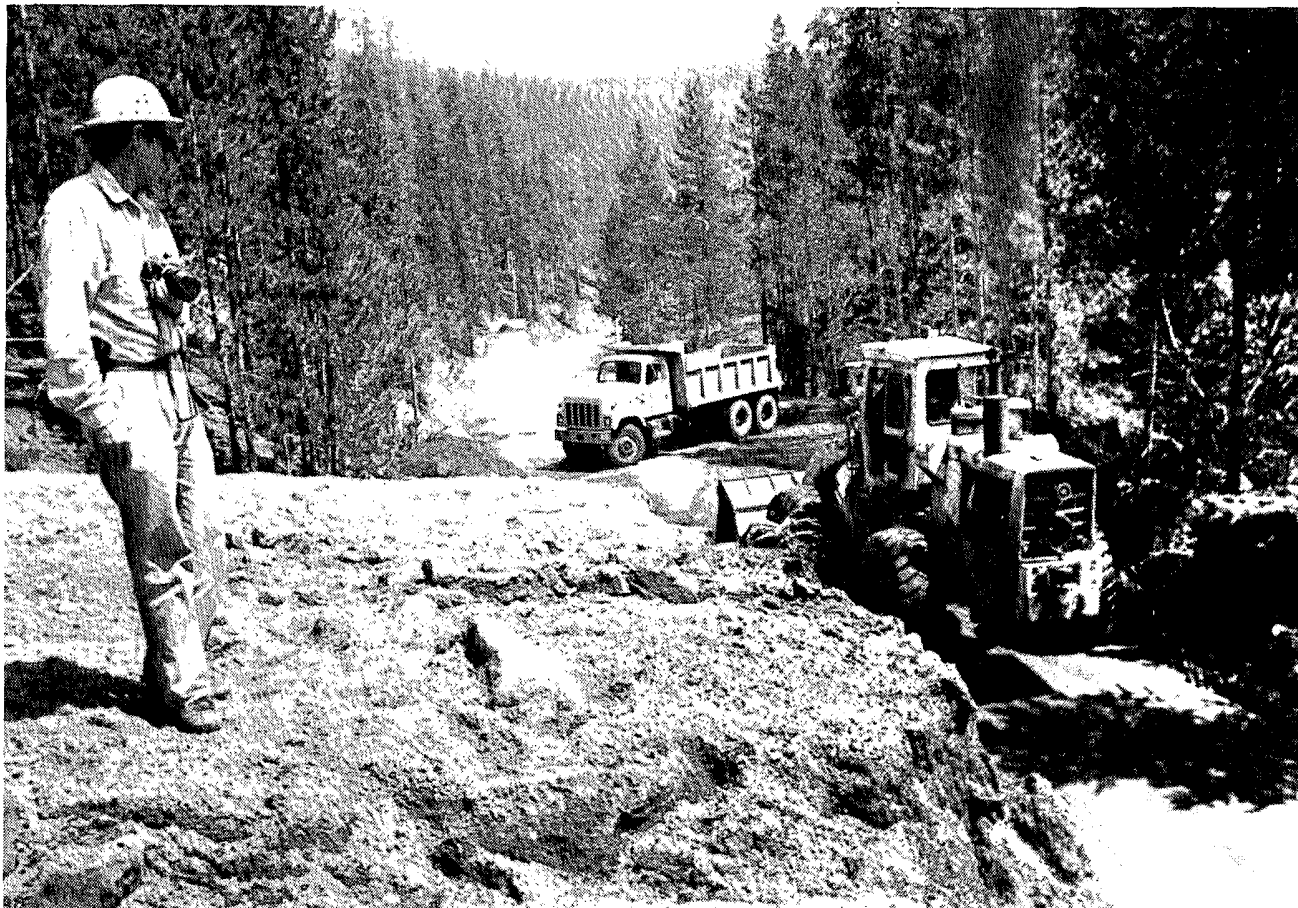
An engineer supervises the removal of slide debris from the roadway.
