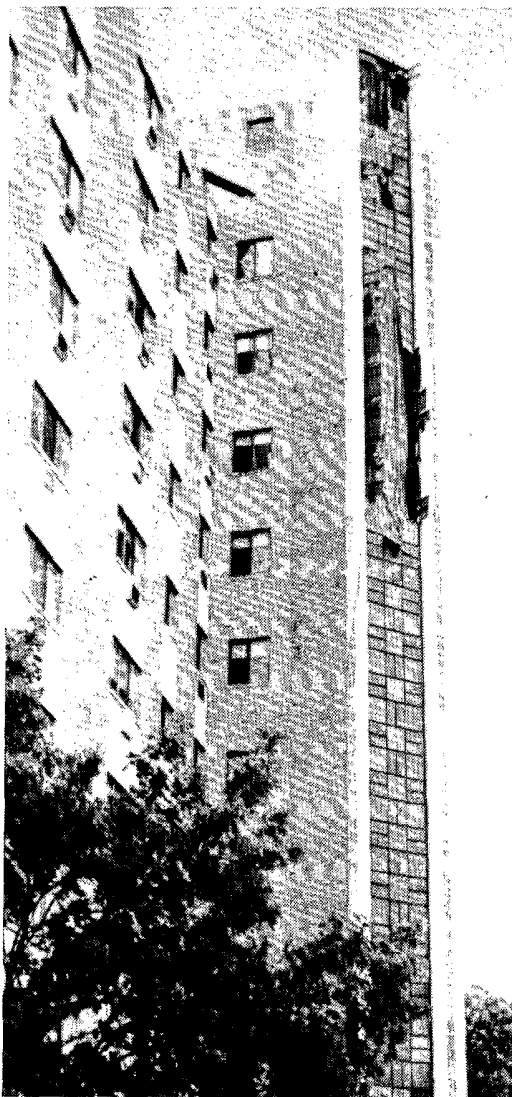
Another heavily damaged structure was this 10-story building near the end of the damage path. The building is the home of Sundial, housing for the elderly.
