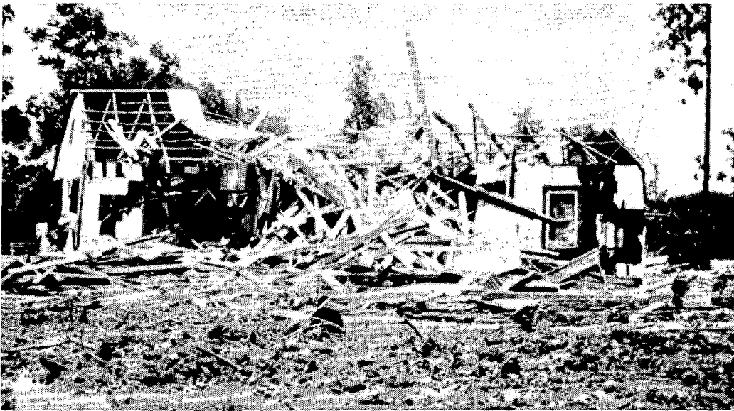
A destroyed home in Grosse Tete. ---Both above photos are by Kenneth Barrick.
