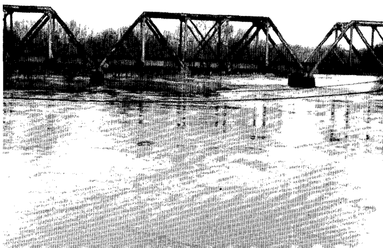
Above, water of the Salt River scales the piers of the L&N railroad bridge at Shepherdsville, Kentucky, the Bullit County seat about 15 miles south of Louisville. Right, onlookers view the high water from a highway bridge in Shepherdsville. ---Both (JR)
