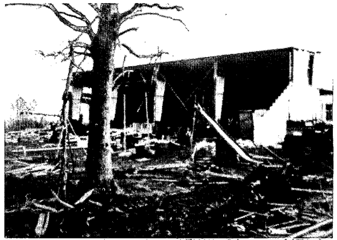
The front, west face of the Allendale school (left) and the north wall of the school's gymnasium (right), located on the north side of the school's main building. The gym's wall appeared to have been yanked off by the winds, whereas the roof stayed in place. ---Both (UI)
