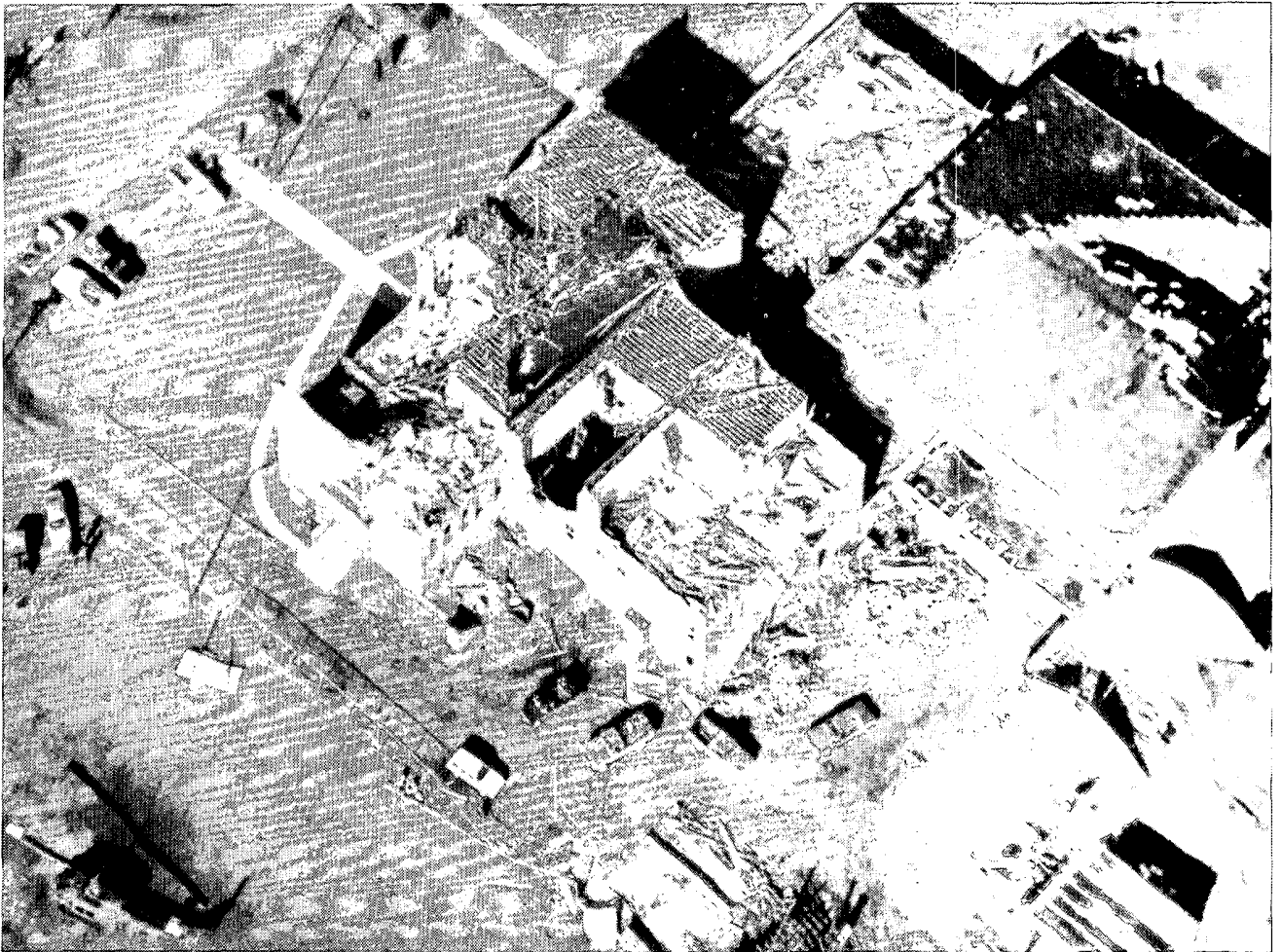
Two aerial views toward the north show the Allendale school from different elevation angles. The school, at the east end of town at the terminus of Main Street, was situated at the south edge of the line of heaviest damage. The building lost much of its roofing and a number of second-story walls. Most windows were broken and there was extensive damage done to the interior. ---Top (BD), bottom (DS)
