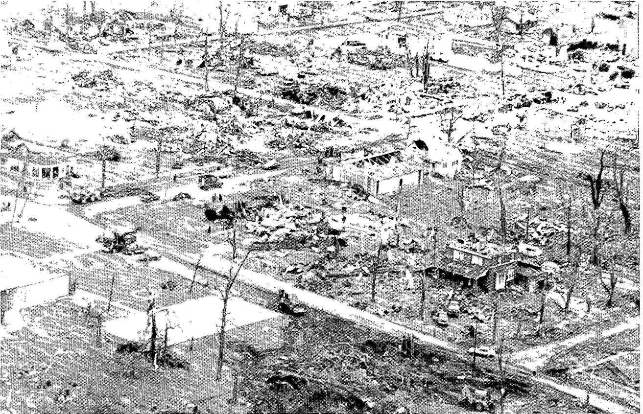
Looking southwest along the line of heaviest damage, this view shows Main Street cutting across the center of the photo, a portion of the town's business district appearing in the upper right corner and the Allendale school in the lower left. ---(BD)
