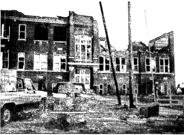
The front, west face of the Allendale school (left) and the north wall of the school's gymnasium (right), located on the north side of the school's main building. The gym's wall appeared to have been yanked off by the winds, whereas the roof stayed in place. ---Both (UI)
