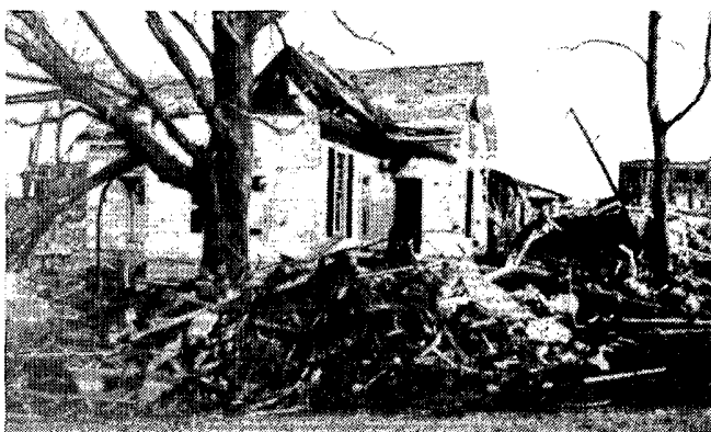
A home across Main Street from the Allendale fire house that was heavily battered by flying debris. The fire house was completely destroyed. On the right in the background is the Allendale school, one block to the east. ---(UI)
