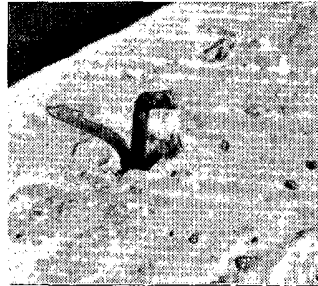
Clockwise from upper left, examples of the anchoring bolts used on the Galliat homes included only the threaded anchor without a nut or washer, one with a nut and small washer that failed to hold and bent under the stress, a threaded anchor without a nut that was merely hammered over onto the bottom board of the wall frame during construction - the wall ripped away anyway, leaving the bottom board on the foundation - and a similarly hammered over anchor from which even the bottom board had been pulled away. ---All four (JS)
