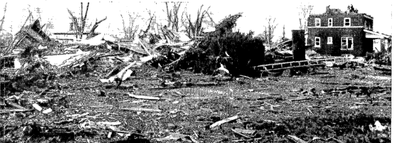
A northward view of another house across the street from the school, this one on the north side of Main. It was demolished by the tornado. The next house to the north, the brick structure at the right edge of the photo, lost its roof. ---(UI)
