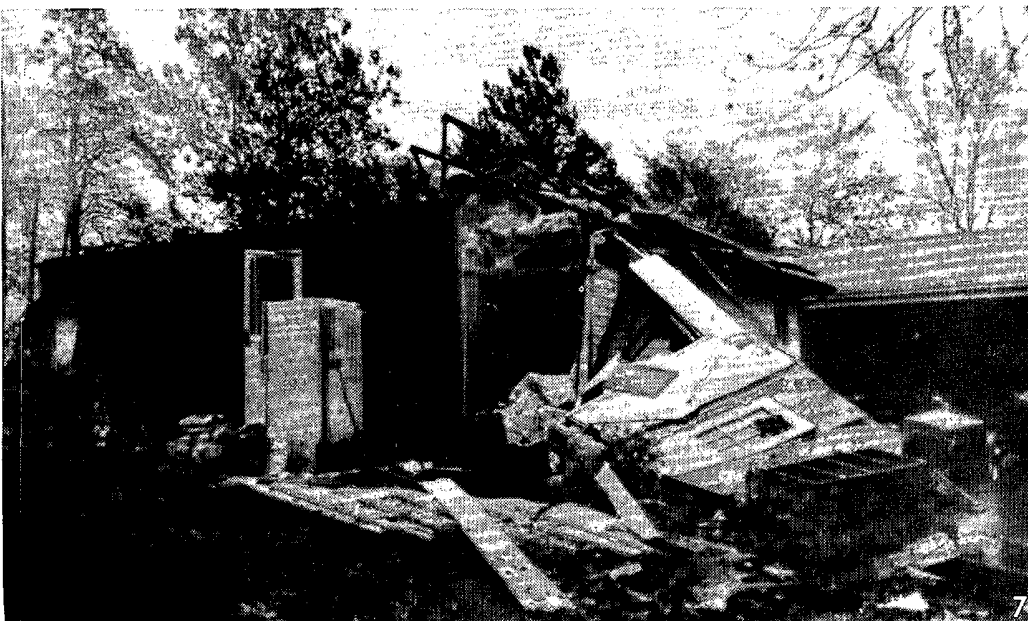
As was determined from the pattern and intensity of their damage, the two homes above, located side by side along the south side of County Road 48 between County Roads 9 and 11, were probably struck by a suction vortex that came at them from the northwest as it spun around the backside of the parent tornado. The westernmost home, viewed toward the southwest at top, received roof and siding damage as it was most likely clipped by the vortex, while the other home, viewed toward the southeast, had extensive damage done to its west half, on which the vortex would have scored a direct hit.
