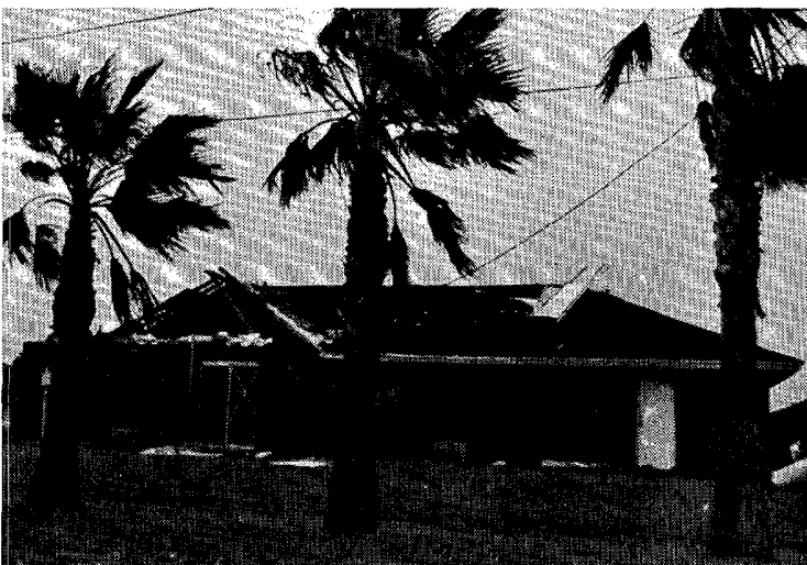
Roof damage to a Harlingen home. Unbroken were sliding glass doors just beneath the damaged section of roof which had been taped in anticipation of GILBERT's winds along with all of the windows in the house.
