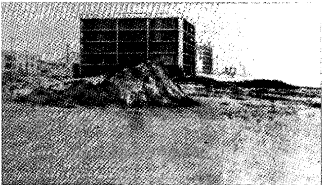
Dune erosion along the Gulf shoreline in South Padre.
