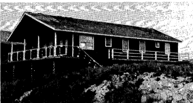
Roof shingle damage on a beach house in South Padre.
