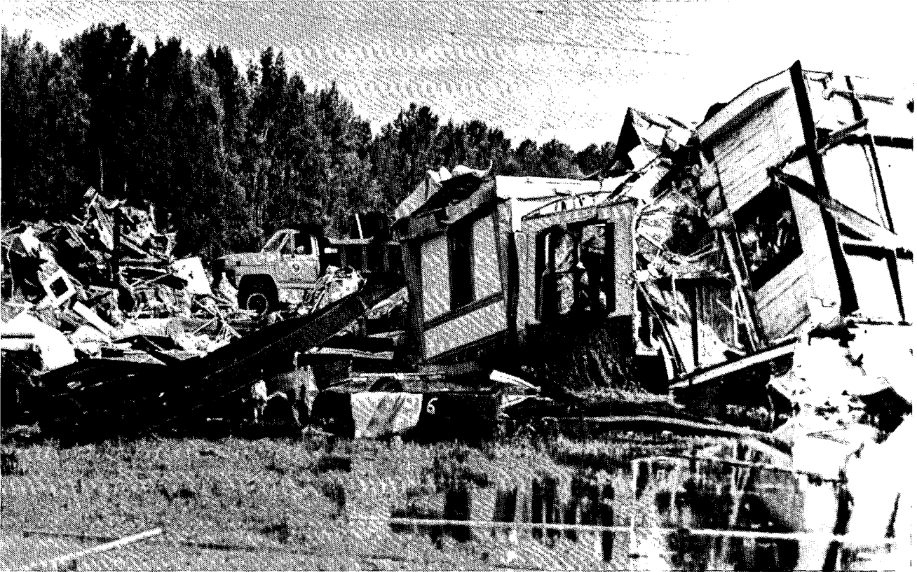
Many of the mobile homes as above were rolled into each other forming trailer sandwiches, while for others (foreground) only their frames remained intact.
