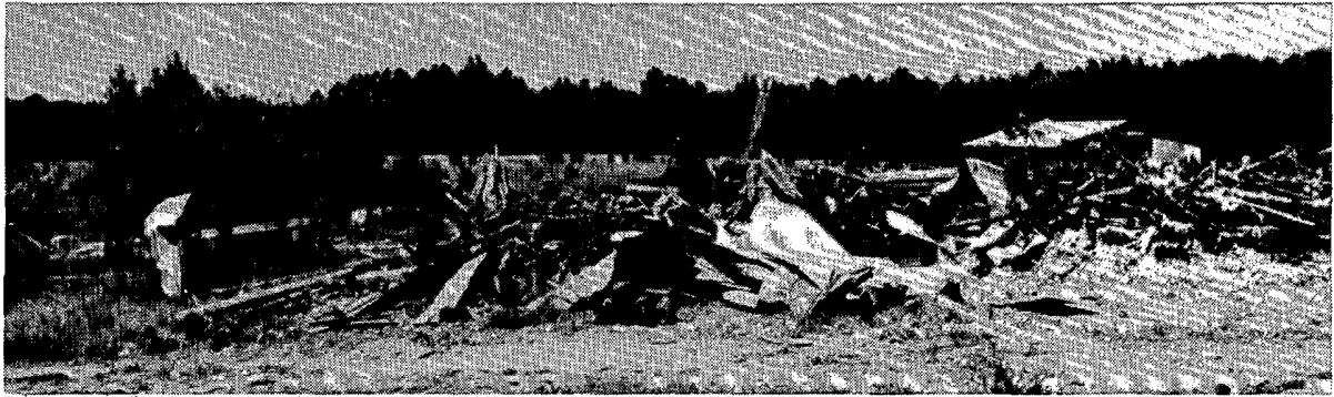
This pile of rubble is all that remained of two barns near State Highway 49 after the tornado destroyed them.
