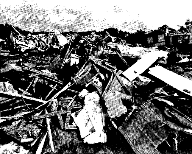
Debris that was gathered into large piles during the removal of salvagable items from the wreckage.
