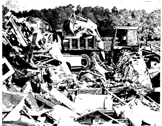
A cleanup crew employs a backhoe to load debris onto a dump truck for removal.
