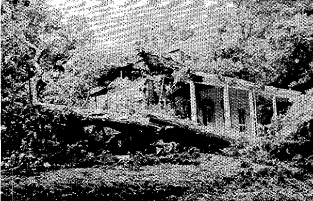
A downed tree and the damage it produced to a home in Lakeside, a north suburb of Richmond.
