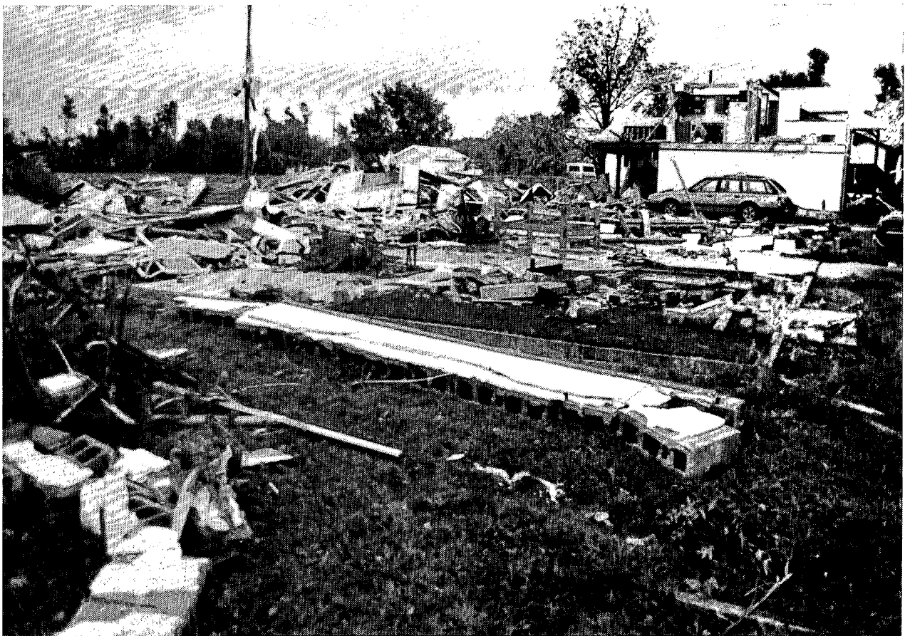
Two foundations (foreground) and scattered debris are all that remain of the Nusser home and a neighboring residence on Avenue K; an adjacent home (background) also received heavy damage. ---(SG)
