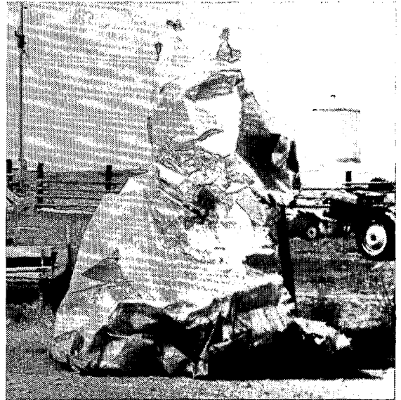
An employee of the Williams Brothers Hog Farm examines a large grain bin (left) that had been moved about 75 feet from its base (right). The bin was about 75% full when hit. The farm, about 3 miles northeast of the IX Ranch, was struck by the first, middle tornado of the three in the area at the time (see map on page 8). ---Both photos (NWS).
