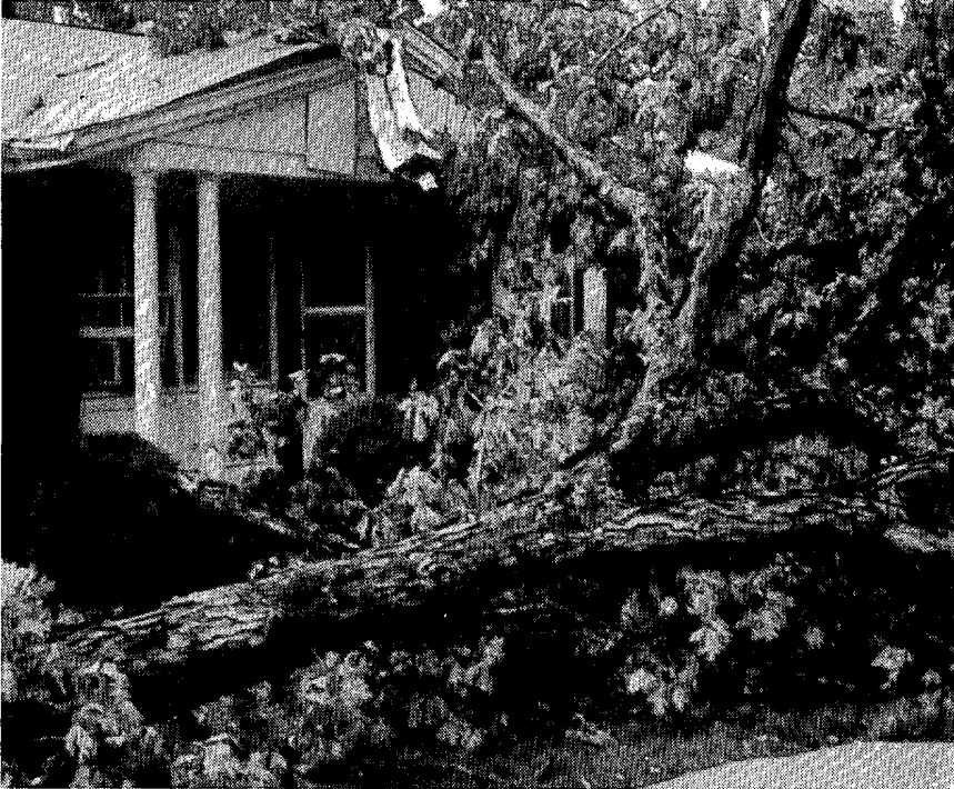
The downed tree blocks the entryway to the home. The offending branch entered the roof above the entryway and poked through the ceiling just beyond the front door.
