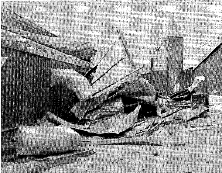
An employee of the Williams Brothers Hog Farm examines a large grain bin (left) that had been moved about 75 feet from its base (right). The bin was about 75% full when hit. The farm, about 3 miles northeast of the IX Ranch, was struck by the first, middle tornado of the three in the area at the time (see map on page 8). ---Both photos (NWS).
