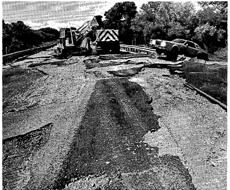
Three closer views of the road damage on Texas Highway 16 at Mercer Creek. The auto left hanging on the guard-rail was under water for at least 5 hours, as was noted by a volunteer helper who arrived on the scene after the vehicle was swept in and subsequently prevented other drivers from accidentally entering the hazardous waters.
