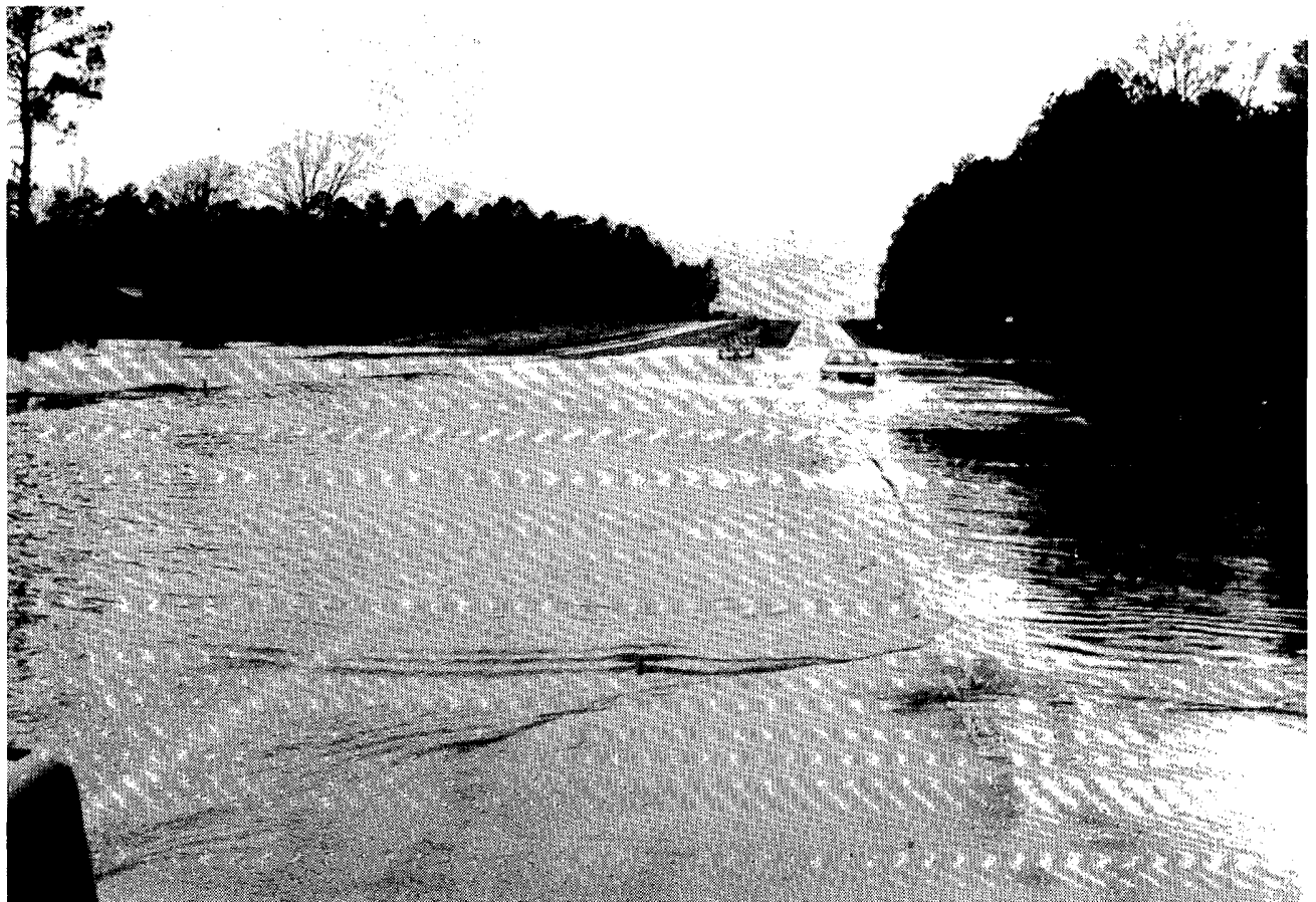
One of two locations on U.S. Highway 190 between Basile and Eunice that were under water.
