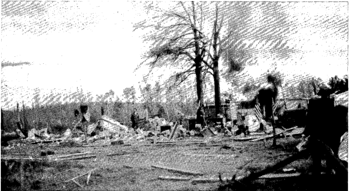
The site of a three bedroom wood-frame home that was cleaned off its cement slab by the tornado. The site is the same one shown in the aerial photos on the previous page. Upon hearing the tornado warning, the resident went next door to stay with her parents, so no one was in the structure when the tornado hit. ---(NWS).
