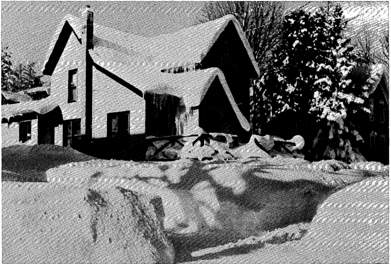
Following the storm, a rather large accumulation of snow adorns the roof and yard of this Lyons Falls home. Note the large icicles hanging from the home's eaves.
