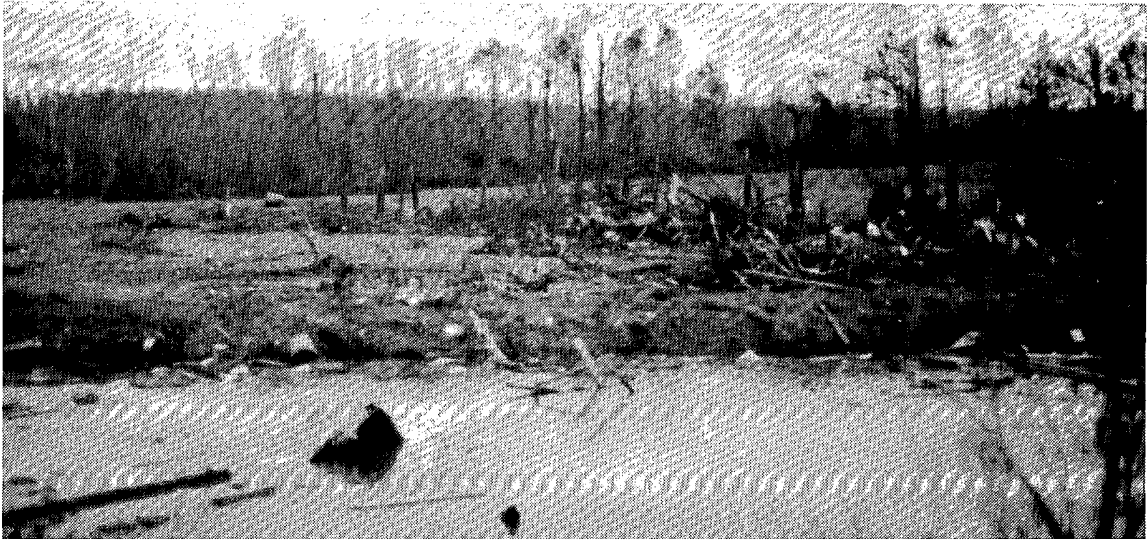
Just northeast of the previously pictured site, debris from the house is seen spread out over several hundred yards. ---(NWS).
