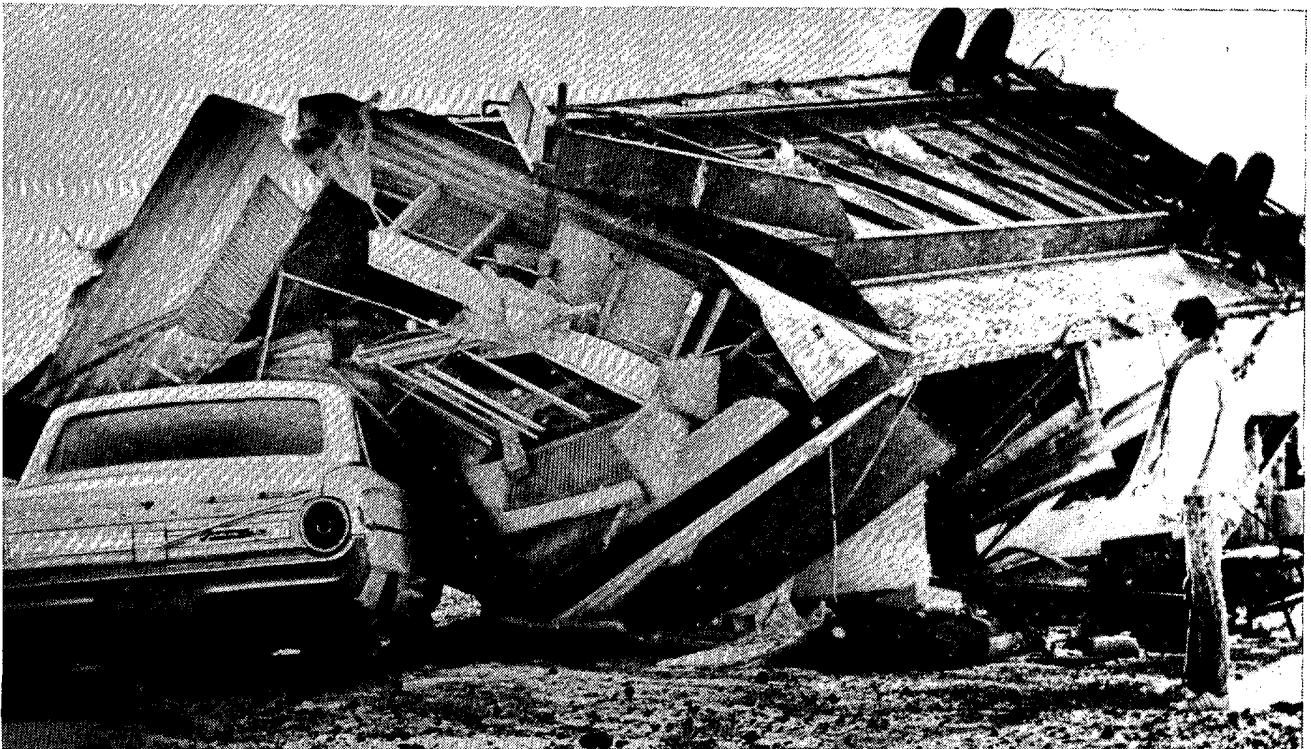
A mobile home in the Gillette, Wyoming area that was flipped over by wind gusts on January 24th. The home landed atop one car and was stopped from rolling farther by another car and a fence not seen in the photo. ---Photo by Kathy Novak, The News-Record, Gillette, Wyoming; and supplied by Hugh McRandal, NWSFO at Cheyenne, Wyoming.
