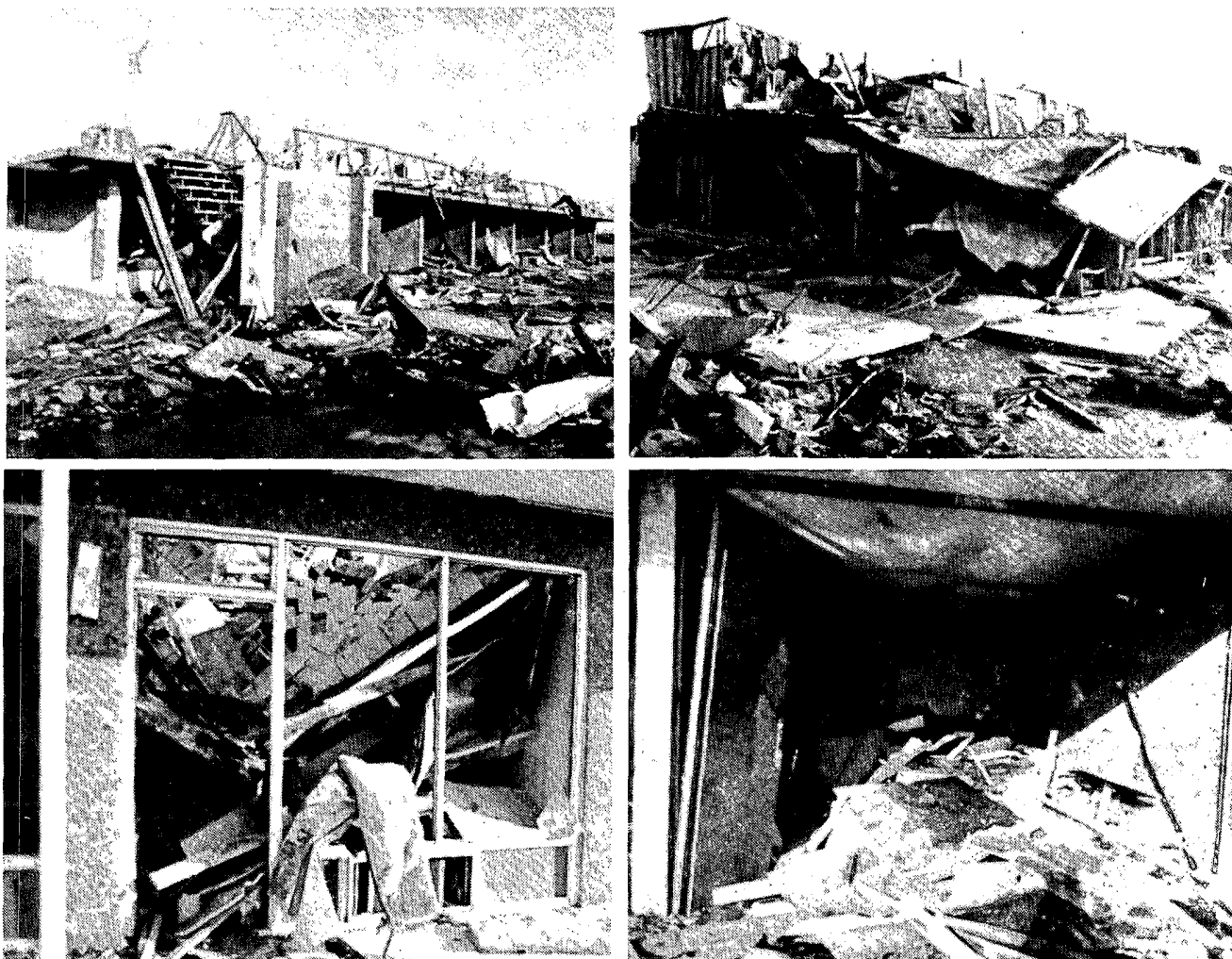
11-14. Four views of the destruction sustained by the Scottish Inn, a two-story wood and masonry structure with a lightweight concrete roof, located on the south side of Interstate 40. The second floor was completely destroyed while the lower level received irreparable damage. At lower left is a second-story firewall that had fallen through the floor and into a first-story room. Miraculously, no one was killed at the motel.
