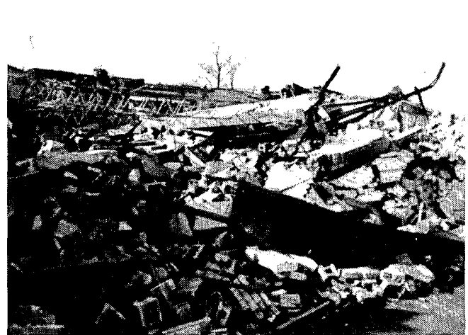
5. Wreckage of unreinforced masonry walls that collapsed at a grocery store at Broadway Boulevard and 15th Street. A teenager caught outside in the store's parking lot was killed when struck in the head by flying debris.
