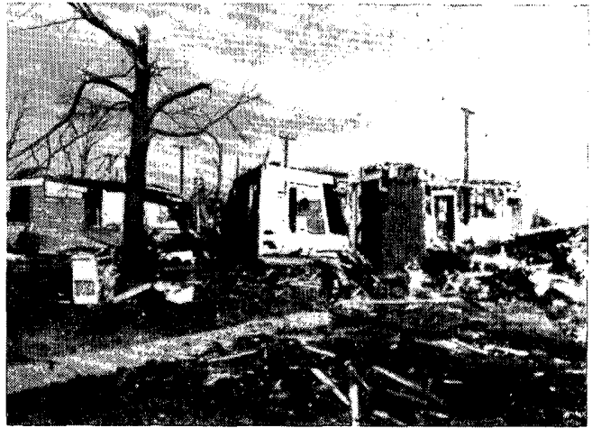
9. A well-constructed brick home that lost its roof and a few of its exterior walls.
