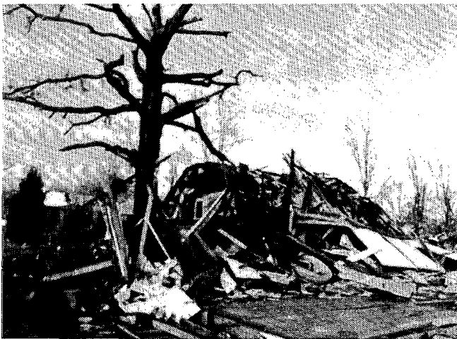
2. Remains of an old wood-frame house near 8th Street and Jackson Avenue. Many of the homes in this old and impoverished neighborhood experienced similar fates, but some were merely shifted off their supports while remaining intact.
