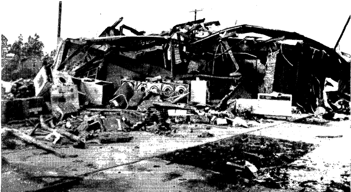
10. Twisted remains of a light steel frame, strip shopping center that had its windward wall pushed in. This portion of the building housed a laundromat.
