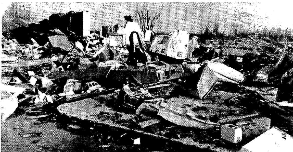
15. A liquor store along Interstate 40 that was levelled.
