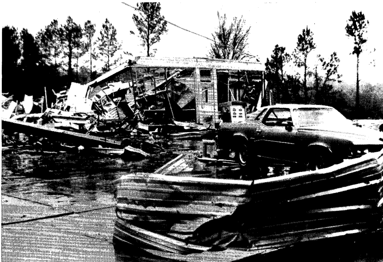
A destroyed gas station/store along U.S. Highway 171 at the southern edge of Shreveport. Three people in the store hid under a desk when the tornado struck, after which it took two hours to free them. One person who did not make it into the store hung on to a nearby telephone pole and watched as two horses from a barn 250 yards southwest of the store flew by. ---Photo by Jack Barham, The Shreveport Journal.
