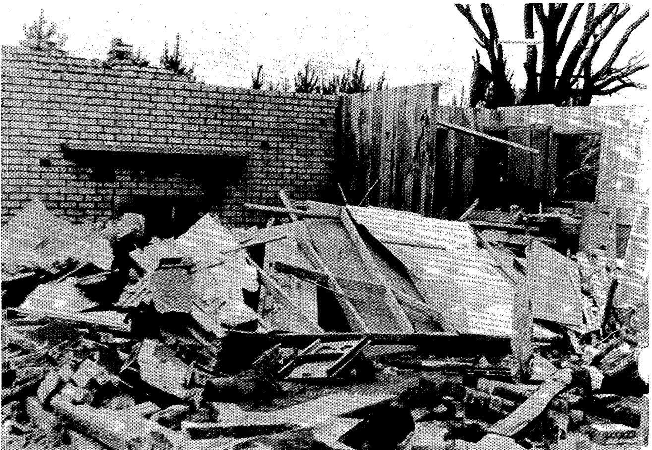
Exterior and interior views, top and bottom respectively, of a brick house that was destroyed by an F3 tornado near the Cross Roads community, southeast of Marietta in northwest Cass County, Texas. Three persons sustained injuries at the site. ---Both photos from The Monitor, Naples, Texas.
