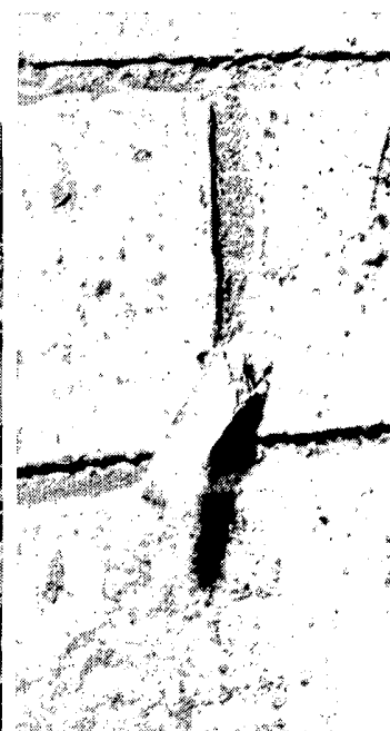
One injury occurred when an F3 tornado destroyed this house (left), 12 miles north-northeast of Hughes Springs, Texas. Near the same location, a small piece of wood was driven into mortar between concrete blocks (right) about 150 yards west of the tornado's damage path. ---Both photo from The Monitor, Naples, Texas and provided by Ernest S. Ethridge, NWSO at Shreveport, Louisiana.
