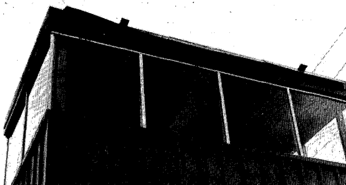
Although minor, damage was also sustained by the National Weather Service Office at the south end of Mueller Airport, demonstrated here by roof flanging that was bent upward on the south side of the building (top) and the north side of the second-floor observation deck (bottom).
