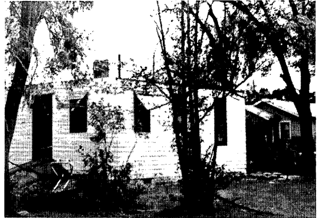
A home that was unroofed by thunderstorm winds at 15th and Grove in northeast Wichita, also on the morning of the 5th.
