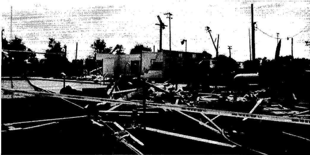
Southwest view of the damage at the public swimming pool located in the city park at the west edge of Morocco. The cement block building (center) lost its roof.
