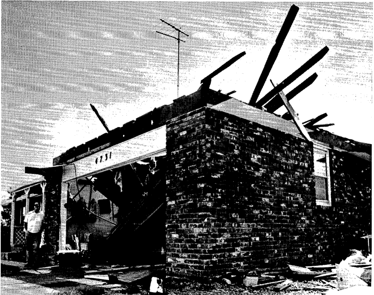
A home southeast of Topeka, Kansas near Berryton, of which the roof of the attached garage collapsed during the strong winds that accompanied the third line of storms that struck Kansas on the morning of the 5th. ---Photo by Steve Wolgast, The Topeka Capital-Journal.
