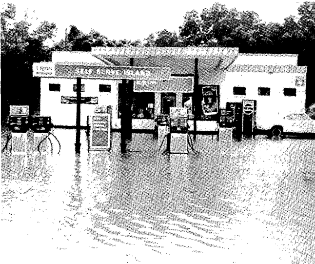
As water climbed the pumps, it certainly was not business as usual at this gas station located along the Goliad Highway (US-59) in Victoria.
