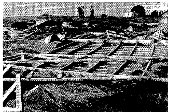
A small barn's roof which was ripped off, carried over a house and mobile home, and scattered across a hay field 155 yards away.
