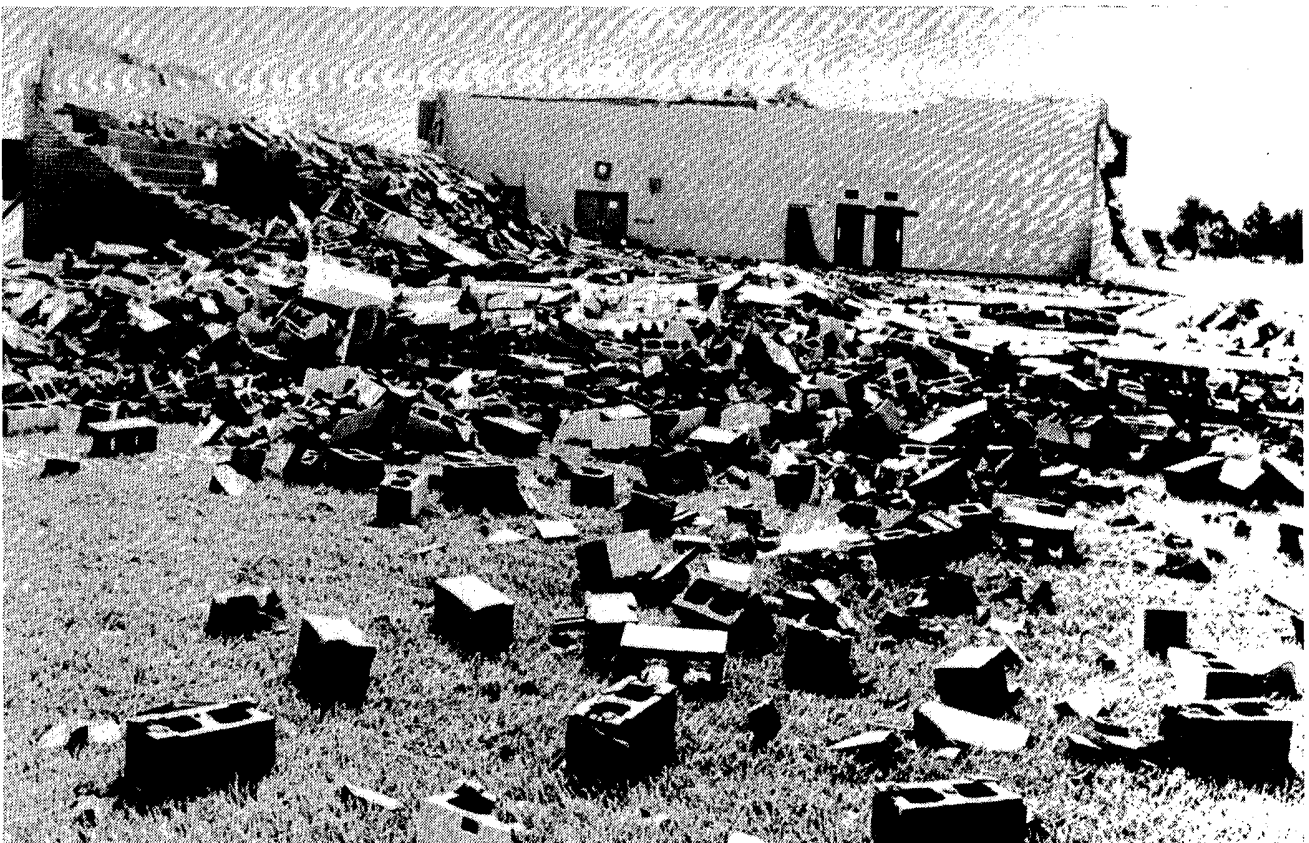
Northward (top) and eastward (bottom) views show the complete destruction incurred by the gymnasium at the North-Central Kansas Vocational Technical School at Beloit. The 99 x 78 foot structure was built about 8 years ago at a cost of $900,000. The attached building is the Student Union which also sustained some damage. ---Both above photos from the Beloit Daily Call; and supplied by Steve Schurr, NWSFO at Topeka, Kansas.
