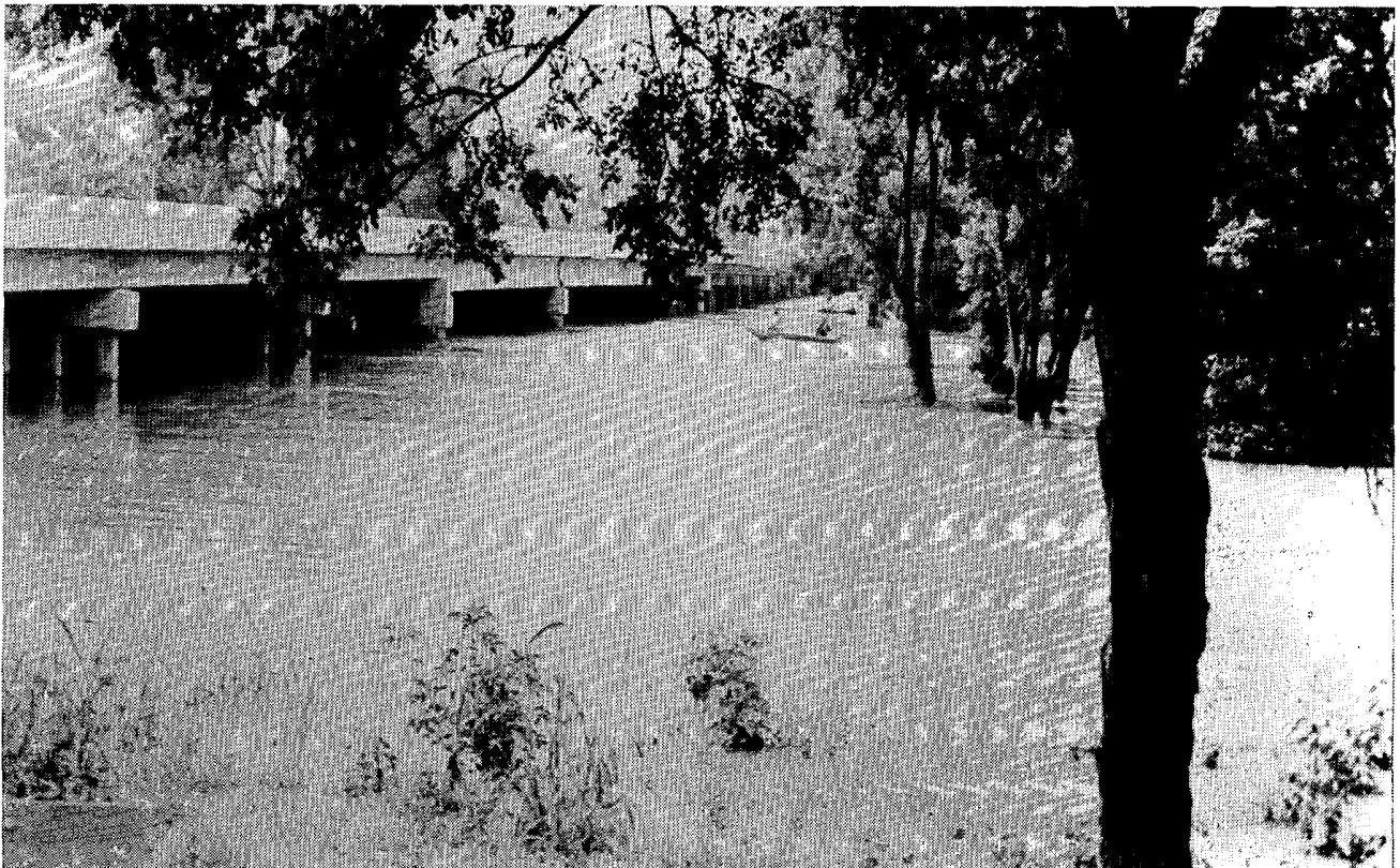
Waters climb the supports of the Guadalupe River Bridge of U.S. Highway 183 south of Gonzales on June 4th. At Gonzales, 6.10 inches of rain fell in a 24-hour period ending at 0600CST on June 4th; 5.50 inches on the 3rd, and 5.02 inches on May 29-31.
