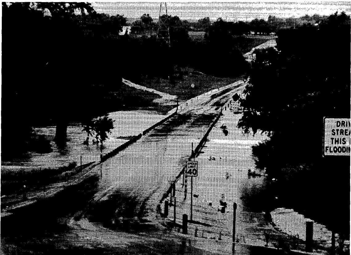
Waters of the Guadalupe River lap at the bottom of the Lemos Street Bridge in Kerrville on June 4th. Subsequent flooding on July 17, 1987 lifted a section of the bridge and piled it against the large Cypress tree at left.
