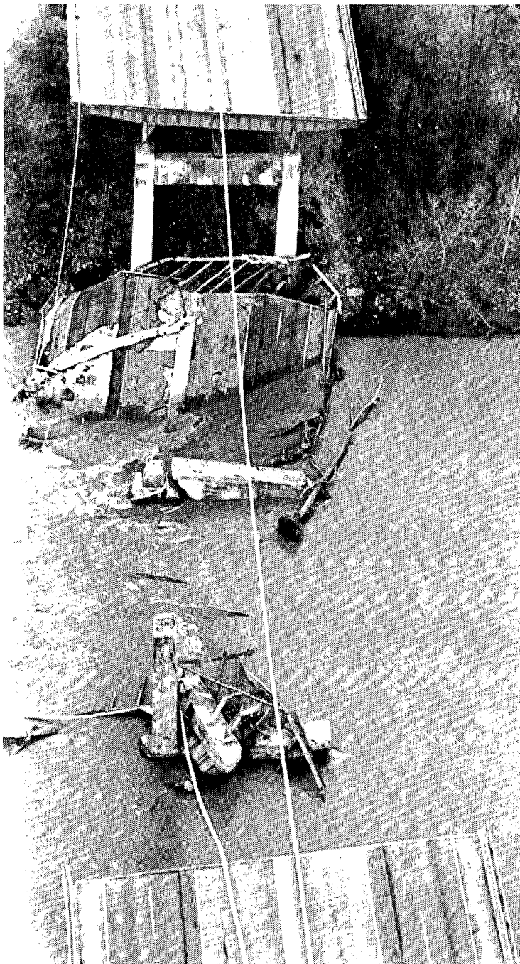
Overhead view of the bridge's crumpled support columns and road surface amid the swirling floodwaters of the creek. Note the median guardrail that still stretches across the void.
