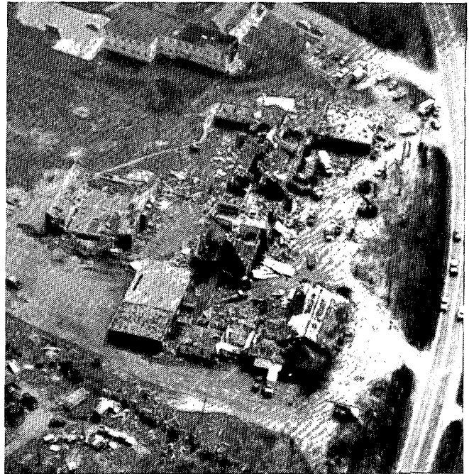
The Glade Elementary School, located across the highway from the water tower, as viewed toward the southeast. The school's main building suffered up to F3 intensity damage, but the detached gymnasium was totally destroyed. ---(UC)
