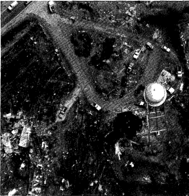
An overhead view of the Glade water tower along Mississippi Highway 15. It suffered only minor damage from impacting airborne debris, while nearby, mobile homes were demolished and practically every tree was felled. ---(UC)
