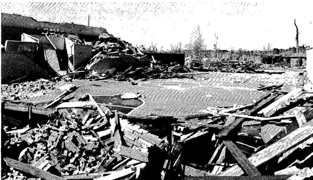
The gym's remains as seen from its east-southeast corner. ---(NWS)
