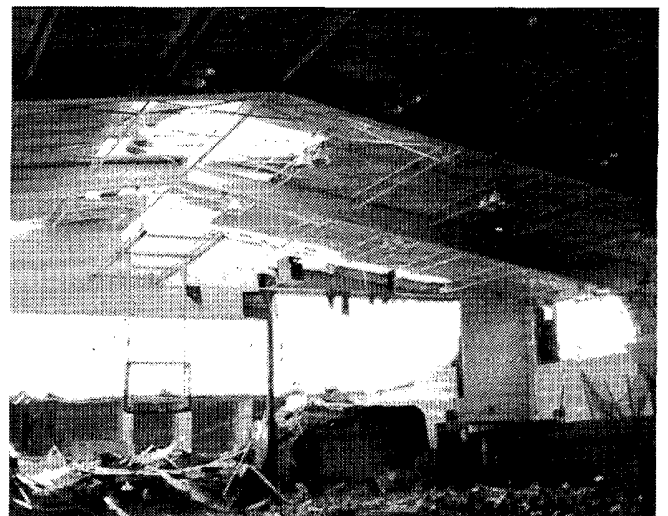
The east end of the hallway of the north wing (left) and the south end of the gymnasium, which collapsed inward, as viewed from inside (right).
