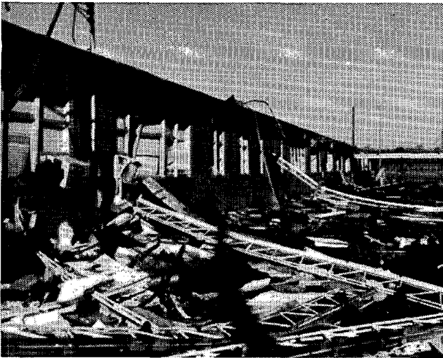
The south wall of the school's north wing (left) and the blown-in windows of the first classroom at the southwest corner of the south wing (right).
