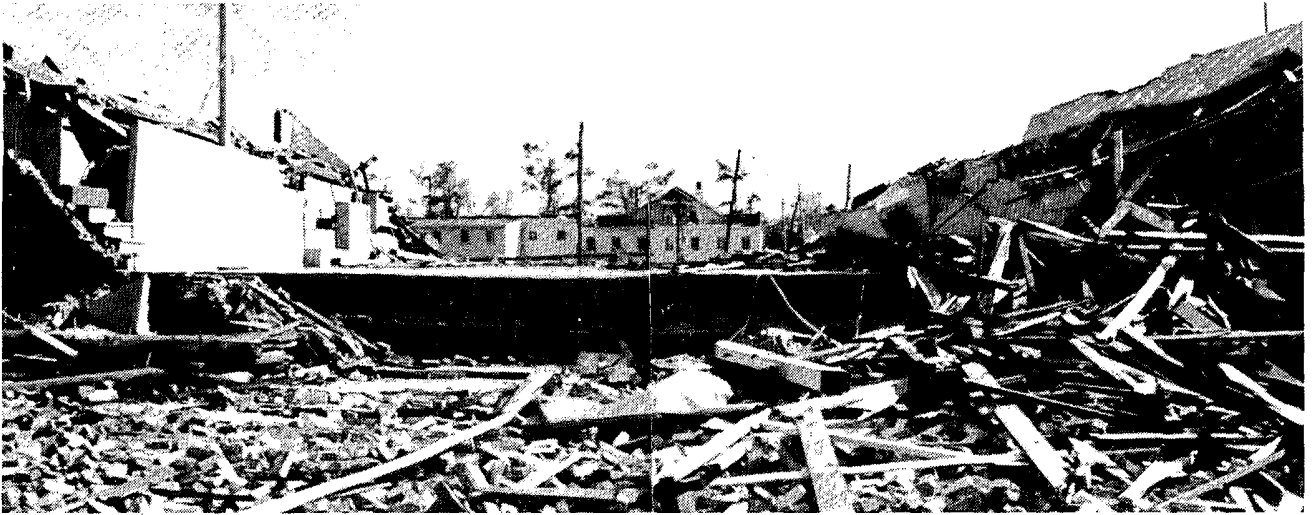
A composite, south-southeast view of the Glade Elementary School's gymnasium shows that all that was left standing were the lower portions of the supporting walls which abutted the spectator stands, and the stands themselves. ---(NWS)
