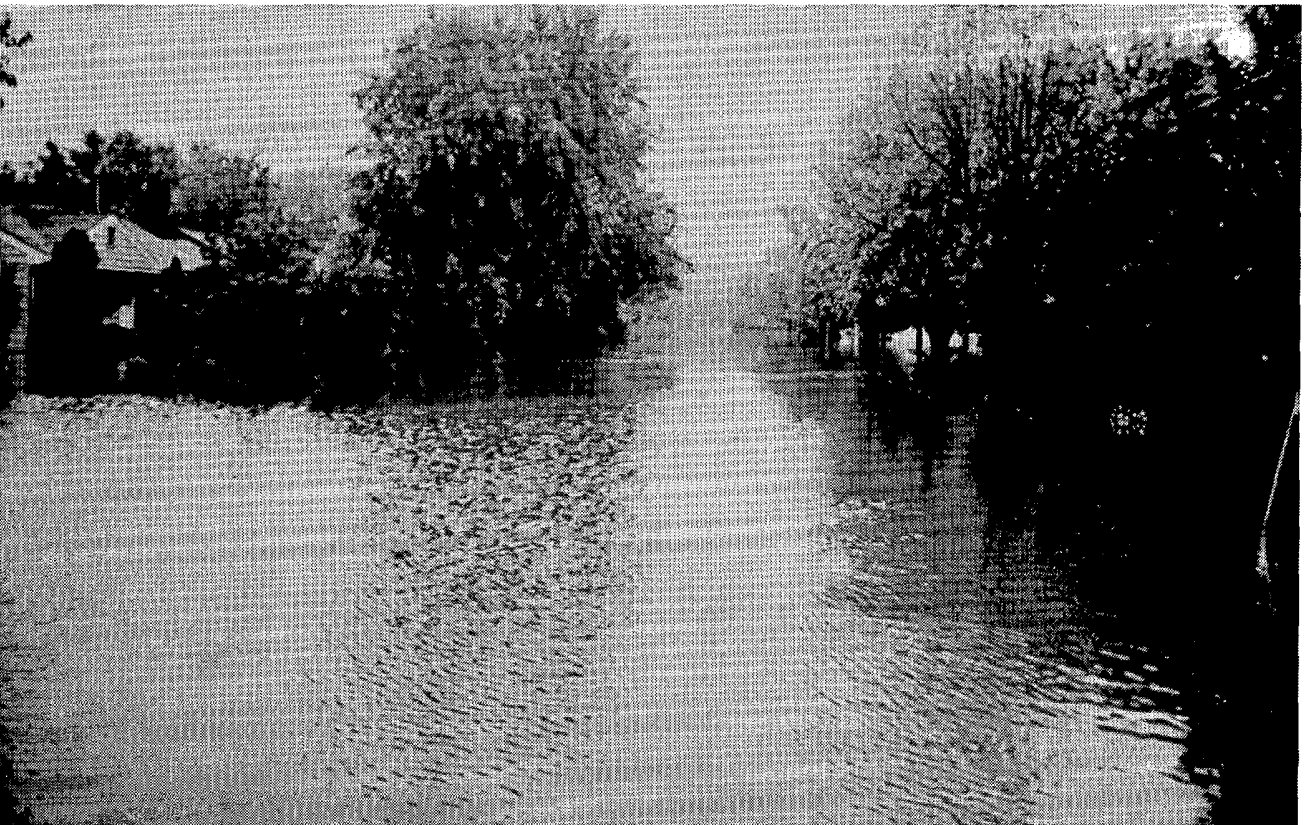
One of many streets of a residential area near Libertyville where almost every home sustained damage. --- (DS)
