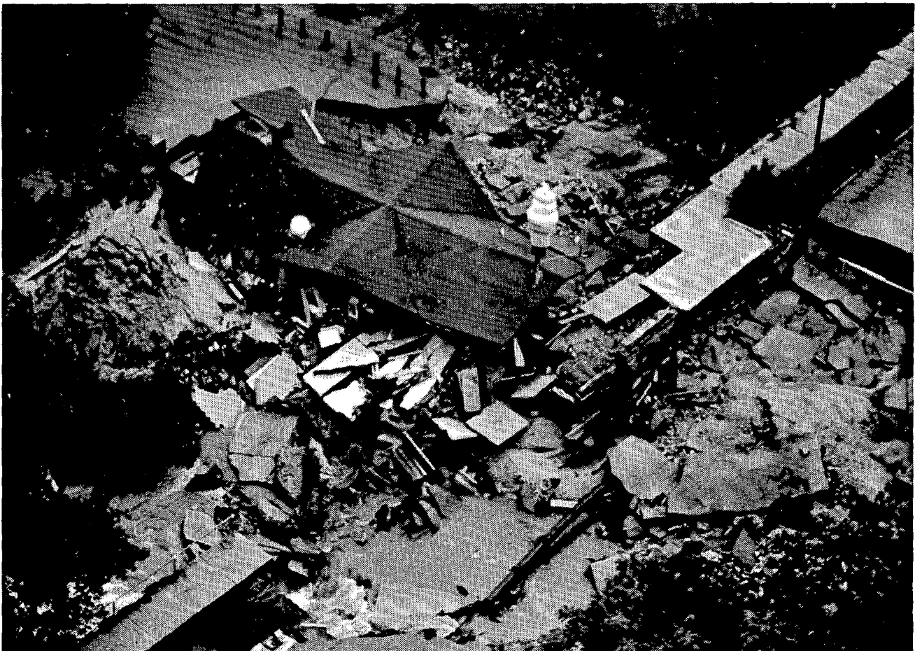
As rains continue to fall, a northwest Grand Rapids resident tries his luck on his flooded street while neighbors tried coping with the unwanted water by swimming and wading in it. BELOW: A Tastee Freeze on Michigan Avenue in Big Rapids that collapsed along with a portion of the street due to erosional forces of rapidly running water in adjacent Mitchell Creek. ---Both photos by Anna Moore Butzner, the Grand Rapids Press.
