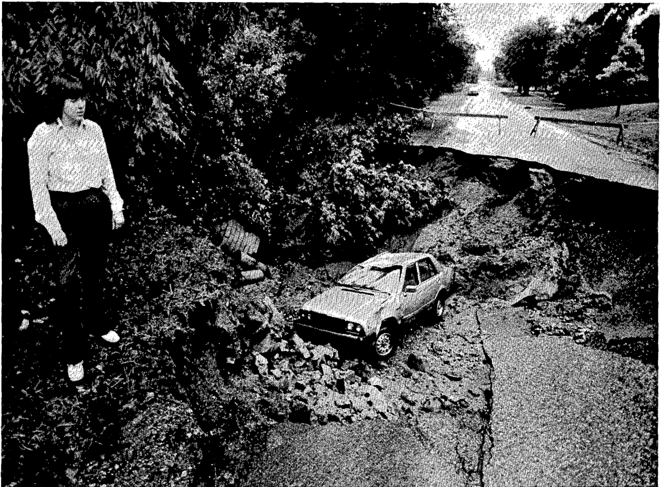
ABOVE: A woman waits for a crane to arrive and lift her car from a huge hole left by the floodwaters in Big Rapids, about 50 miles north of Grand Rapids. 13.13 inches of rain was recorded at the town's waterworks during the deluge. ---Photo by Marvin Laninga, the Grand Rapids Press.
