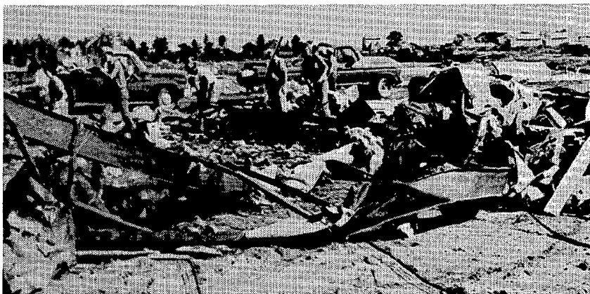
Wreckage at the Jack Clark farm in northwest Republic County. The farmer's house was blown nearly a quarter of a mile east of its foundation. ---Photo by Deb Sheridan, The Belleville Telescope.
