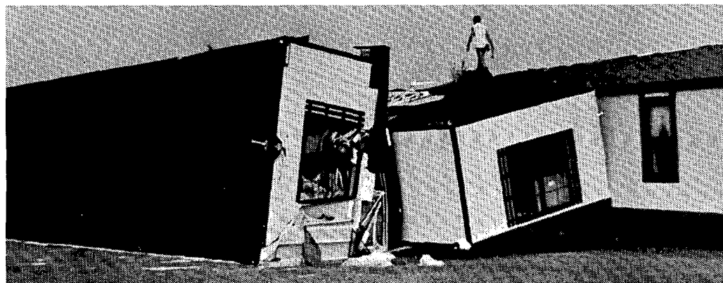
Mobile homes east of Iola that were rolled by the winds. They were at a dealership and hence, not tied down. ---Photo by Bruce Symes, The Iola Register.
