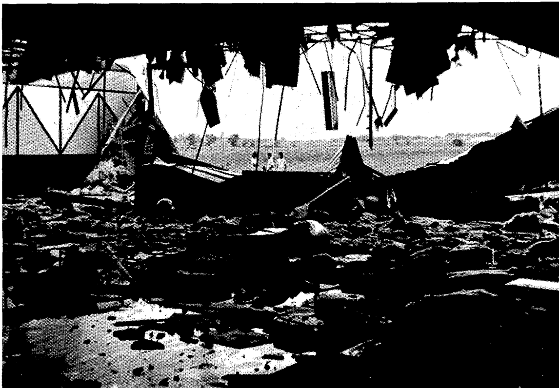
A skating rink east of Iola that had its north wall blown in and part of its roof torn off. ---Photo by Bruce Symes, The Iola Register.
