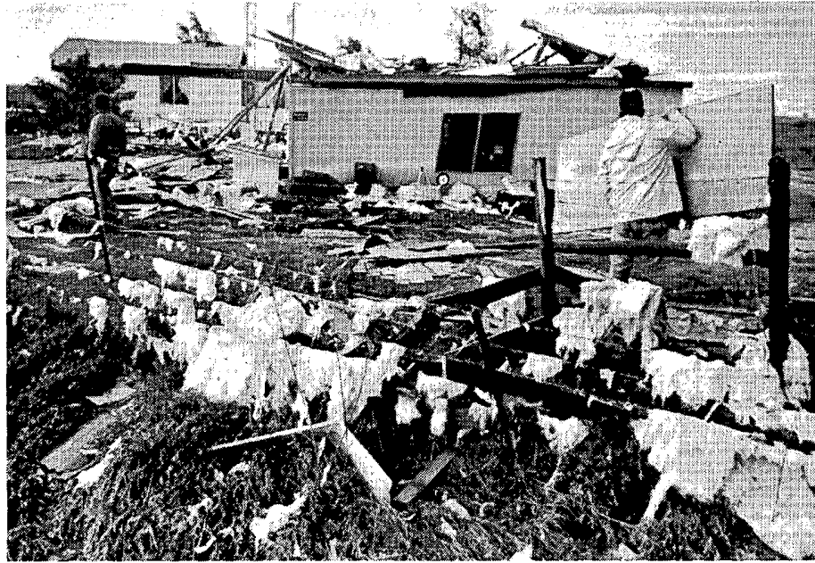
An unroofed home east of Emporia where winds were estimated to have been stronger than 80 mph. ---Photo by Marc Stratton, The Emporia Gazette.
