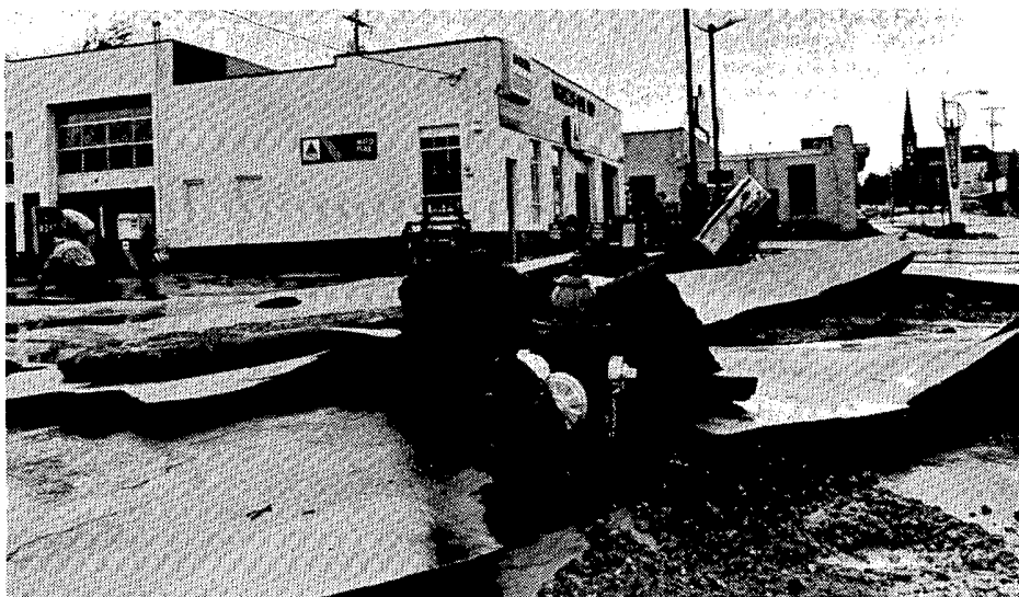
Large pieces of asphalt that were torn up and moved about by the floodwater along Cherokee Street in the downtown area.
