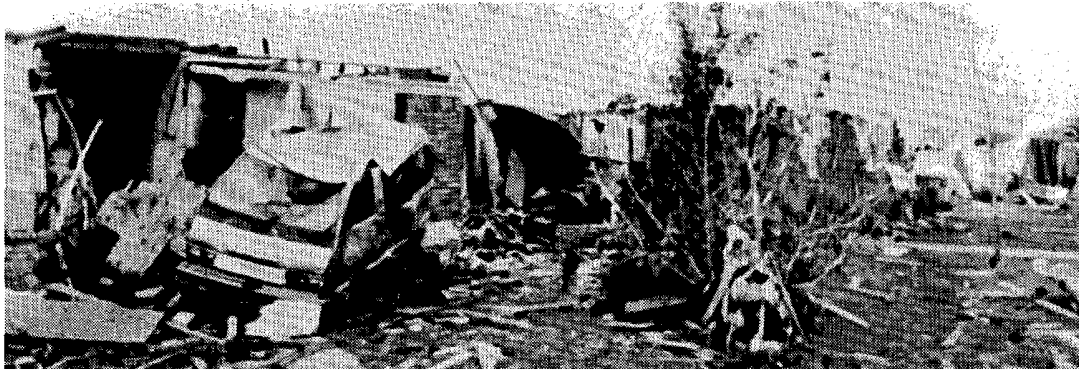
At about 0.25 mile east of the trailer park, these relatively new (less than 5 years old), one story, single-family homes of brick veneer construction received F2 and F3 damage. The vehicle was thrown about 75 feet.
