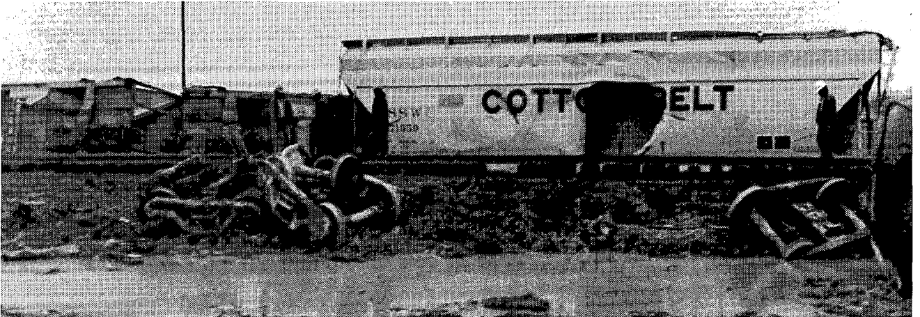
Several of the 28 freight cars that were derailed by an intense, mile-wide downburst as a 130 car train traveled northbound near Penrose, about 20 miles north-northeast of Brinkley. 21 of the cars were empty, and the derailment cost was set at $411,000.
