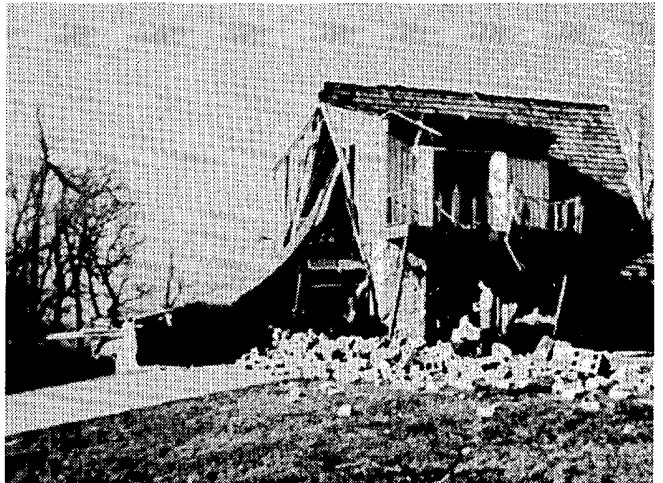
At Continental Manor, located on Lincoln Road about 10 miles NNE of Martinsville, half of this structure (viewed NW) was sheared away by the tornado.
