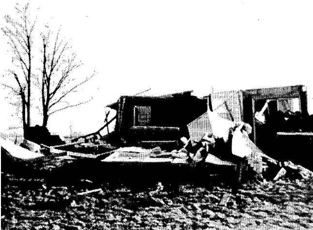
F3 damage sustained by a home located about 14 miles NE of Martinsville (view looking S).
