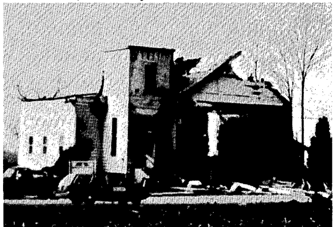
A church (viewed NW) that was unroofed by one of the Fairland Twin Tornadoes at about 4 miles NE of Fairland. Fairland is also along I-74, about 14 miles southeast of Indianapolis.
