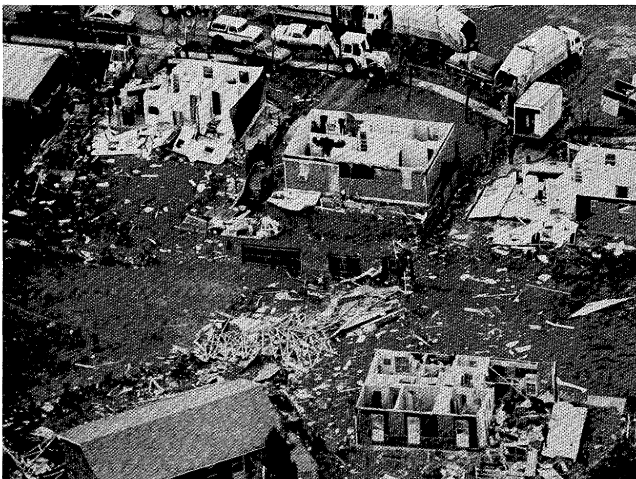
Two aerial views of homes at Ak-Sar-Ben Park which received the tornado's strongest damage, F2 but nearly F3. Almost all of the affected homes were made of modern materials and construction, and were situated in newer subdivisions on the southeast outskirts of the city. ---TOP: (PS&NACE); BOTTOM: David Perry, (LHL).
