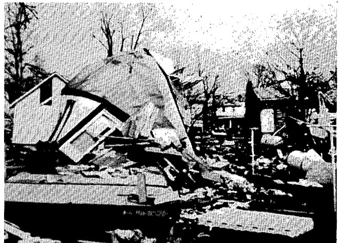
A mobile home at Pleasant View, about 8 miles southeast of Indianapolis along I-74, that was partially twisted from its frame.
