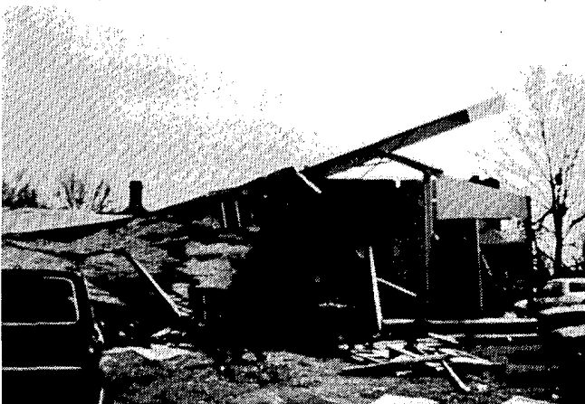
A destroyed service station (viewed E), also in Pleasant View.
