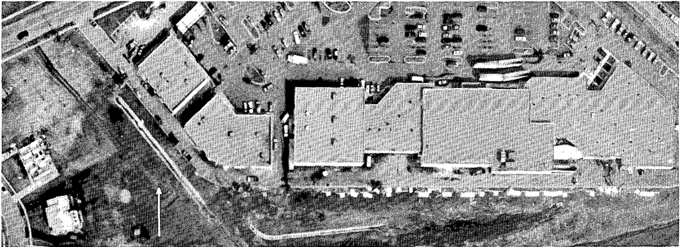
A shopping center near the end of the tornado's path that had roofing peeled and a rear fence blown apart. The house at left was the last to be unroofed. ---(PS&NACE).
