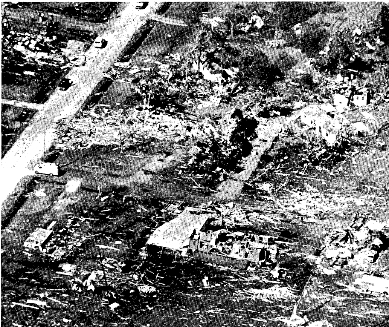
A more overhead view of the Boudreaux Park reveals the chaotic state in which it was left. 37 of 40 mobile homes were damaged or destroyed. ---Craig Hartley, The Houston Post.
