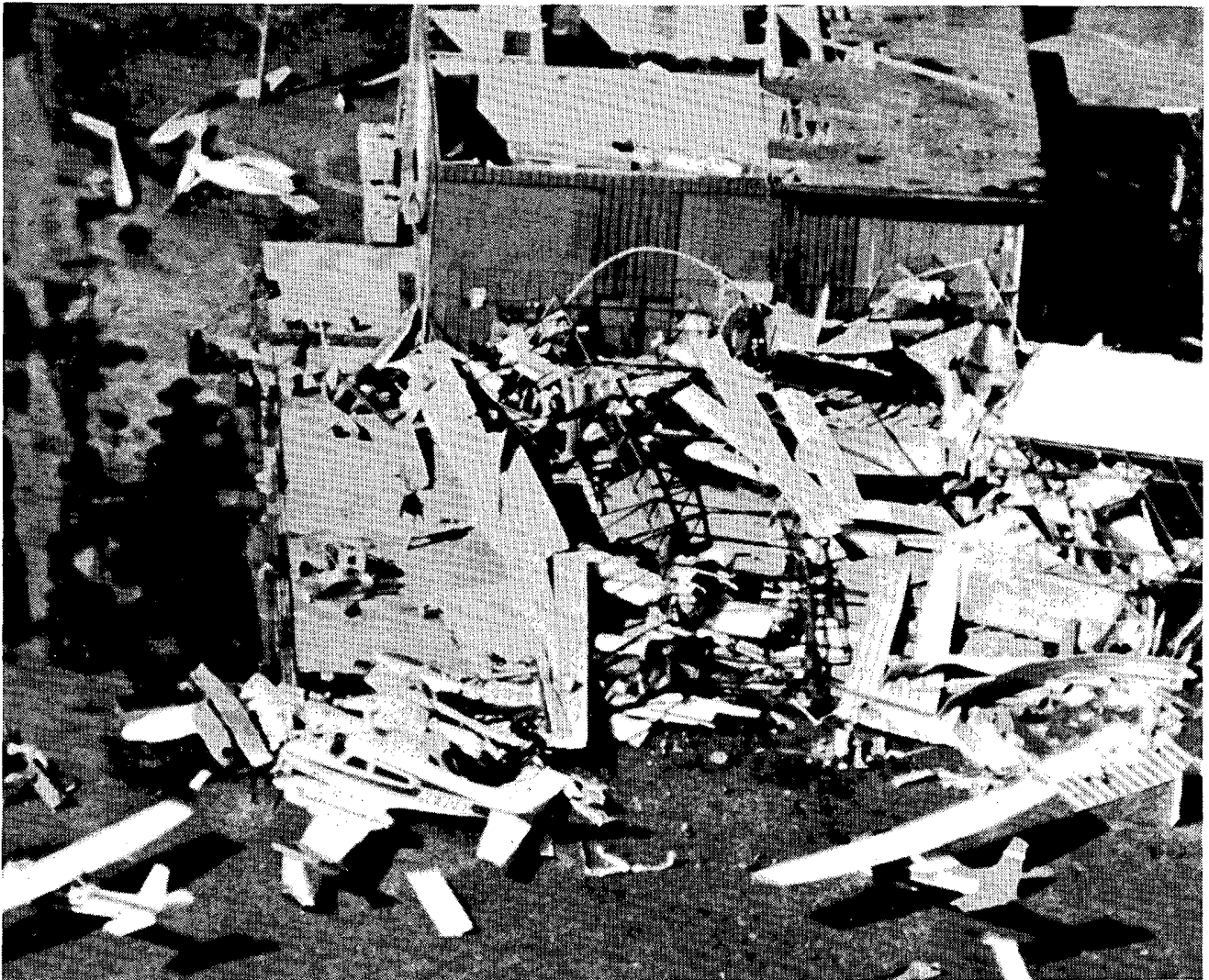
At least 4 planes can be seen pinned under the skeletal remains of this collapsed hangar. The attached office building survived with only a portion of the roof having been removed. ---Craig Hartley, The Houston Post.
