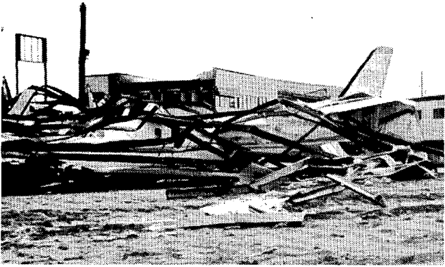
ABOVE: Examples of hangars that collapsed onto aircraft at Hooks. BELOW: Aircraft that were damaged or flipped by diverging winds at Hooks, left, and a plywood missile that was imbedded nearly a foot into the ground at the airport. ---All four photos by Tim Marshall, Haag Engineering Co.
