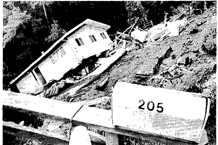
ABOVE: Residents sift for belongings after rain-weakened soil caused this home, once located near the mailbox, to slide down a hill at Fairfax, CA on February 17th. ---Doug Atkins (AP).
