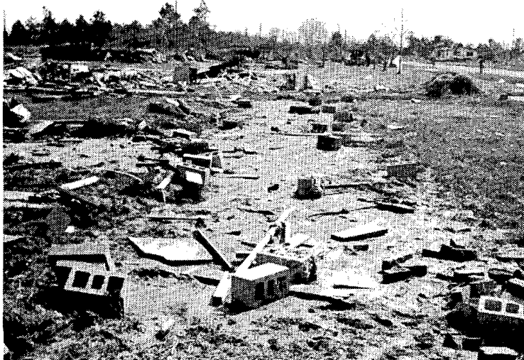
Blocks and broken tie-down straps are all that remain of this trailer at the Boudreaux Park. ---Tim Marshall, Haag Engineering Co.
