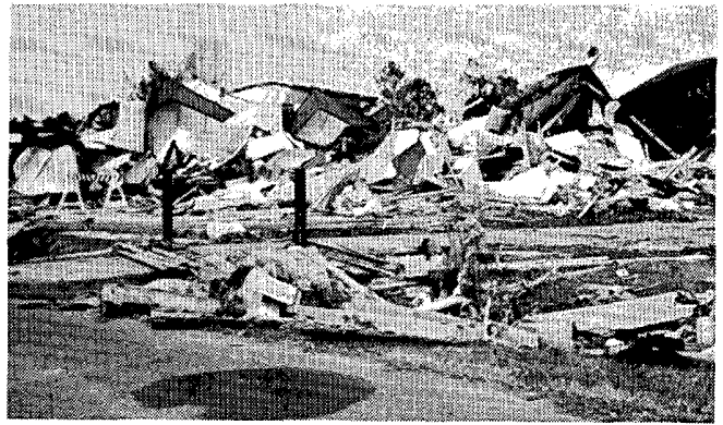
ABOVE: Examples of hangars that collapsed onto aircraft at Hooks. BELOW: Aircraft that were damaged or flipped by diverging winds at Hooks, left, and a plywood missile that was imbedded nearly a foot into the ground at the airport. ---All four photos by Tim Marshall, Haag Engineering Co.
