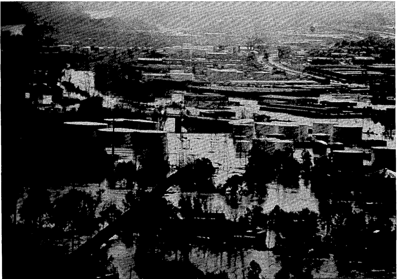
Floodwaters of the James River (foreground) forced the closure of Interstate 95 when they filled the Maury St. underpass (above), and floated petroleum tanks out of position (below). The pictures are side by side views, looking south.
