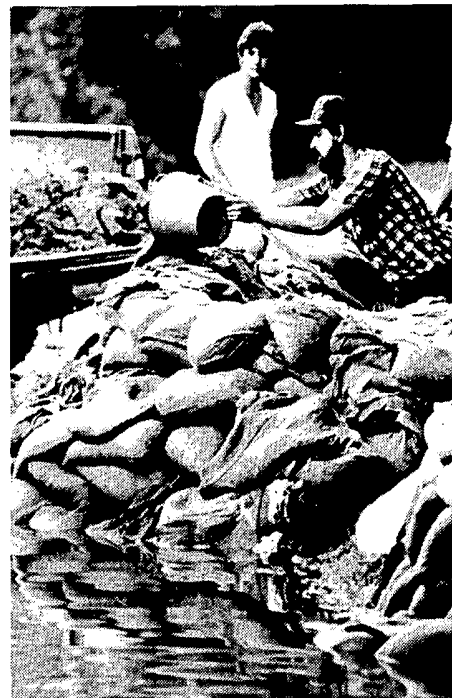
Sandbagging operations which worked well to keep some buildings dry.
