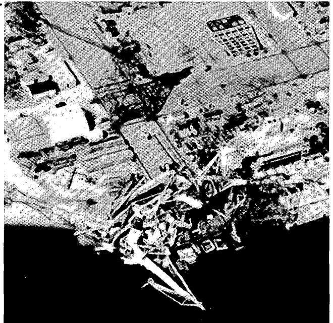
Two cranes that twisted and collapsed around each other at the Ingalls Shipbuilding Yard in Pascagoula. A third, nearby crane survived. ---(DS).
