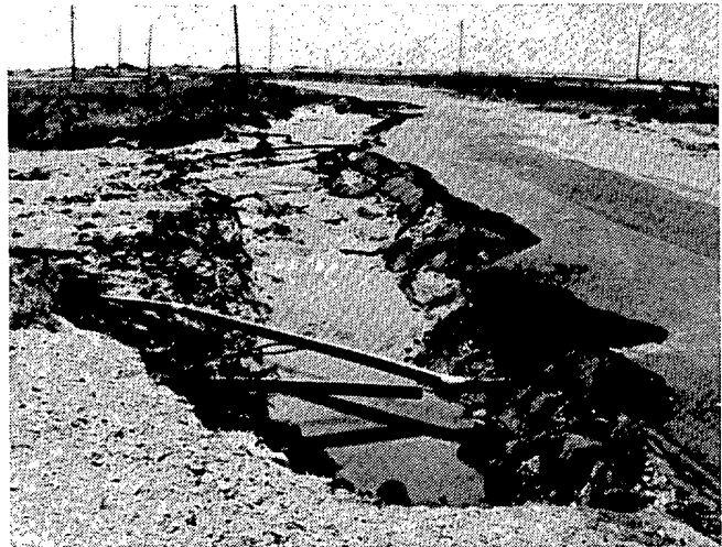
A ground view down the road in the photo at left shows how the sand had to be bulldozed aside to make the road passable.
