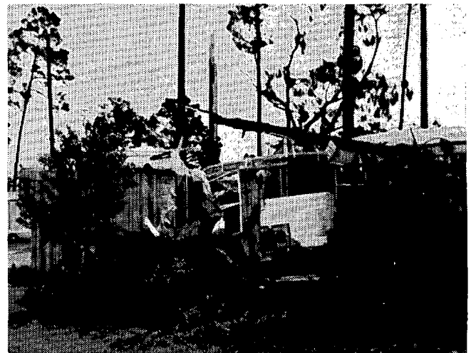
A second trailer at the park that was severed by an uprooted tree. A different, snapped-off tree fell over part of the trailer's roof. ---(BS).
