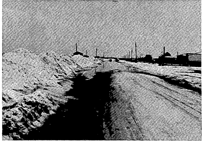
A ground view down the road in the photo at left shows how the sand had to be bulldozed aside to make the road passable.
