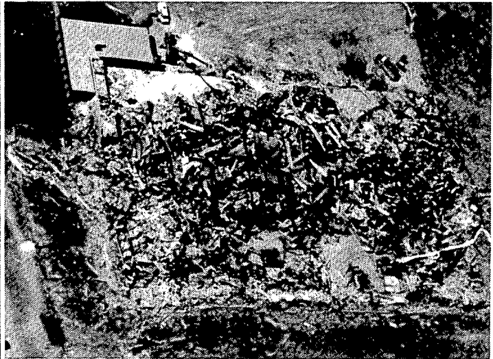
A factory that took a direct hit from the Barrie Tornado in Ontario, Canada.
