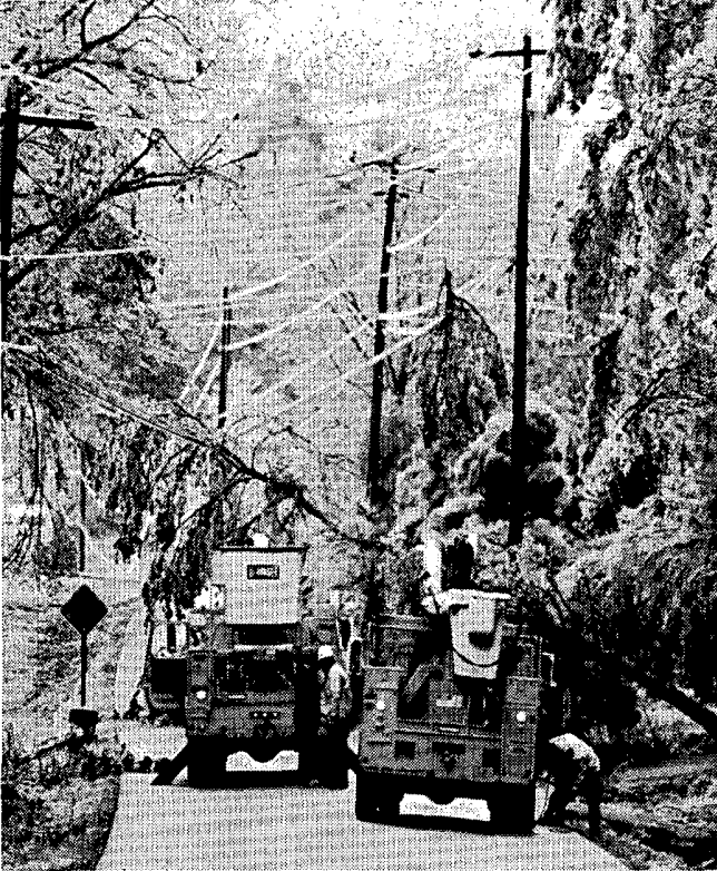
LEFT: Electric crews in Decatur, Alabama are kept busy making repairs to ice-laden power lines that were downed by falling trees and tree limbs. ---Photo by Gary Lloyd. RIGHT: Ice-coated pine limbs litter a Decatur driveway. ---Photo by Glenn Baeske. Both photos from the Decatur Daily.
