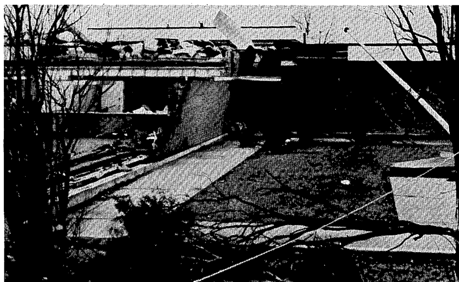
The Potosi Elementary School which sustained loss due to damage estimated at $1,300,000.
