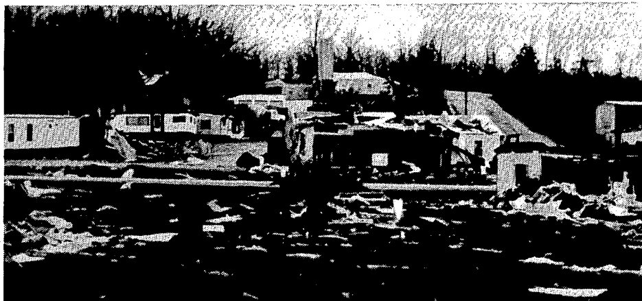
Destroyed and damaged mobile homes at a sales park where the tornado in Potosi, Missouri started.
