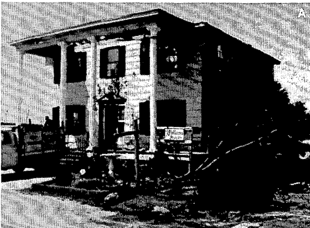
Stagnation pressure, which built up within the portico of this structure in the face of Diana's easterly winds, forced a hole through the overhang, causing a large portion of the roof to be pelted off.
