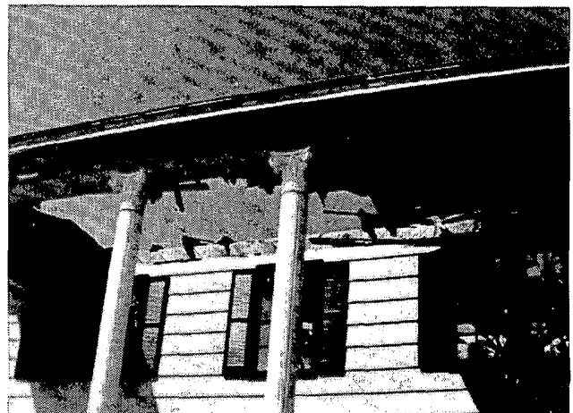
Stagnation pressure, which built up within the portico of this structure in the face of Diana's easterly winds, forced a hole through the overhang, causing a large portion of the roof to be pelted off.
