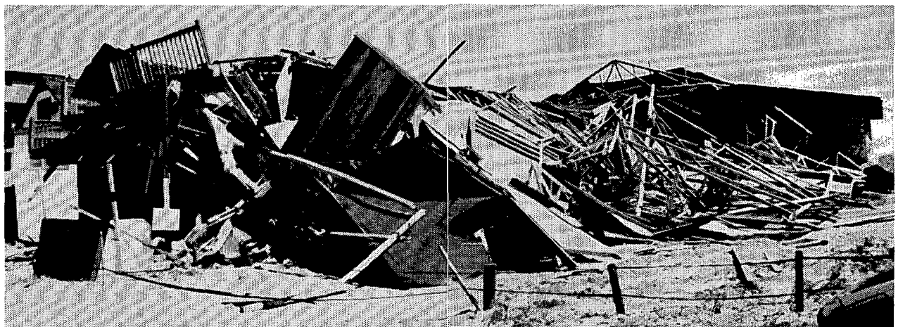
Damage to beach homes and motels in northern Carolina Beach (looking east). Most of the structures received minor roof damage and some water damage. Wind and overwash sent eroded beach sand into homes and streets of the area. The black arrow indicates the view of the photo below, showing a collapsed building that was under construction.
