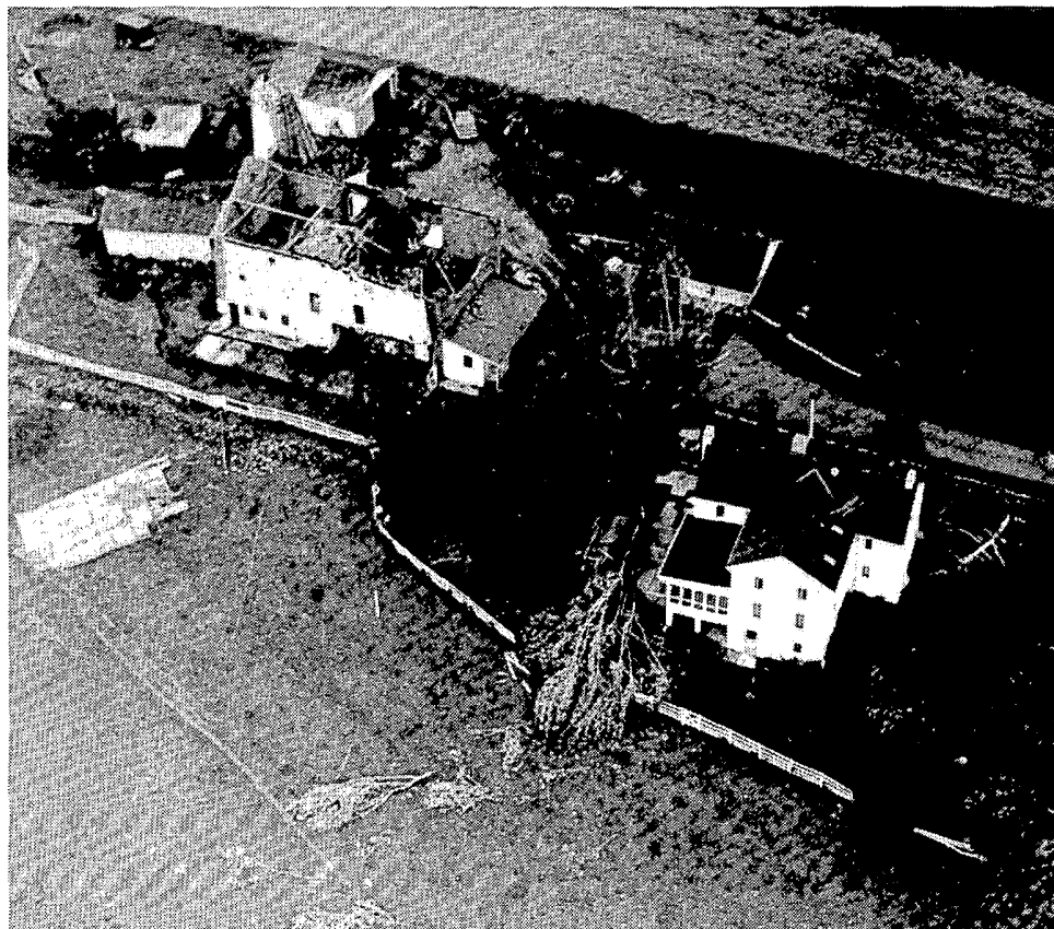
A damaged farmstead within the path of Tornado No. 2.
