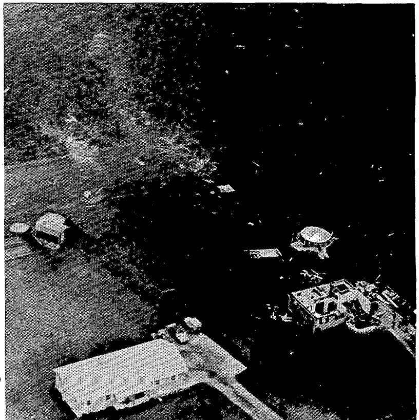
RIGHT: An unroofed home about midway along the path of Tornado No. 1. Note the shed, twisted from its original position.
