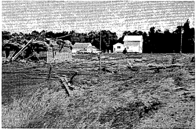
Debris scattered from a wooden barn located 3.5 miles east-northeast of Rowena.
