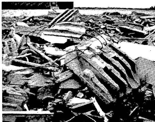
Three views of damage to the Barneveld fire station. The concrete roof was flipped off by the winds, causing it to crumble as it struck the ground. The east, concrete block wall (lower left) also crumbled under the weight of the falling roof. A close-up of a portion of the roof is shown at lower right. Note the cars that were blown into the front of the station. TOP PHOTO: (CT), BOTTOM TWO PHOTOS: (UC)
