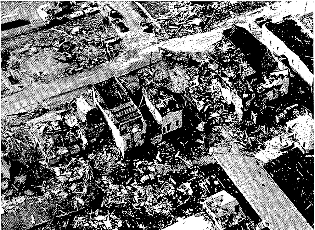
Damage to businesses in downtown Barneveld. (CT)
