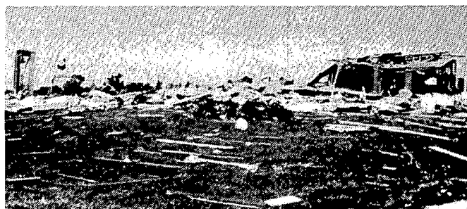
Remains of the Lutheran Church in north-east Barneveld. A car and truck were found inside. (NWS)
