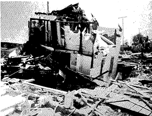
A home that sank into its own basement as it was torn apart by the tornado. (WSC)
