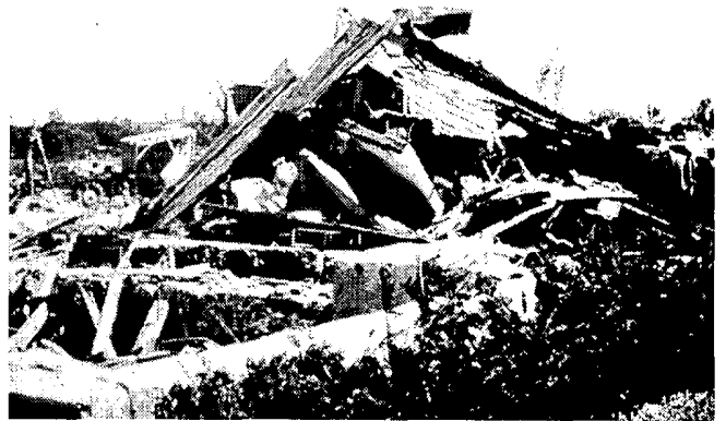
Large sections of this home were left resting in a pile directly behind the foundation. (NWS)
