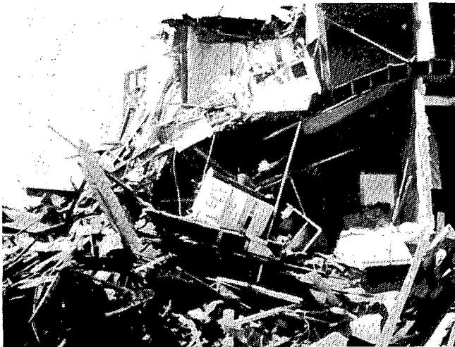
Debris cascades down the front of a two-story building in the business district of Barneveld. (WSC)
