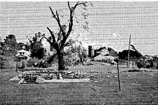
The foundation of a farm home, viewed looking north, where 2 people died. Debris from the house, located 1.5 miles east-northeast of Rowena, was blown northeastward and ended up beyond the location of the electric company truck on the right edge of the photo.
