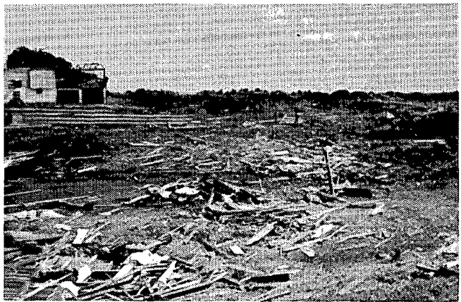
Debris from the home described at left (looking northeast).
