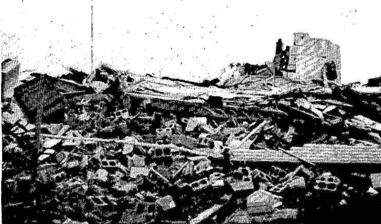
Three views of damage to the Barneveld fire station. The concrete roof was flipped off by the winds, causing it to crumble as it struck the ground. The east, concrete block wall (lower left) also crumbled under the weight of the falling roof. A close-up of a portion of the roof is shown at lower right. Note the cars that were blown into the front of the station. TOP PHOTO: (CT), BOTTOM TWO PHOTOS: (UC)
