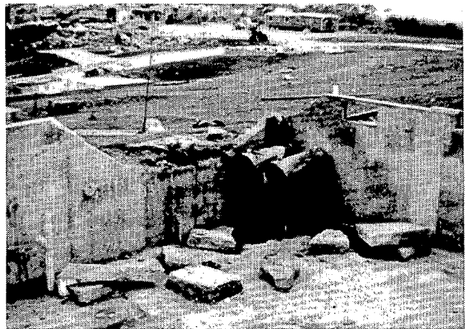
The southwest corner of the foundation of the same home described at left. The wall was broken off by the impact of an airborne object. (UC)
