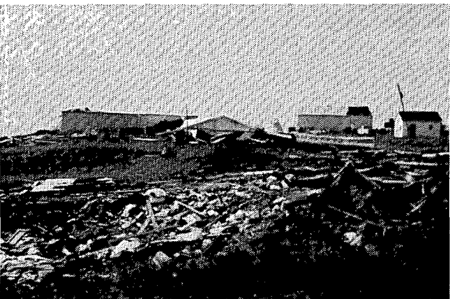
Damage to the rest of the farm where the two people died.
