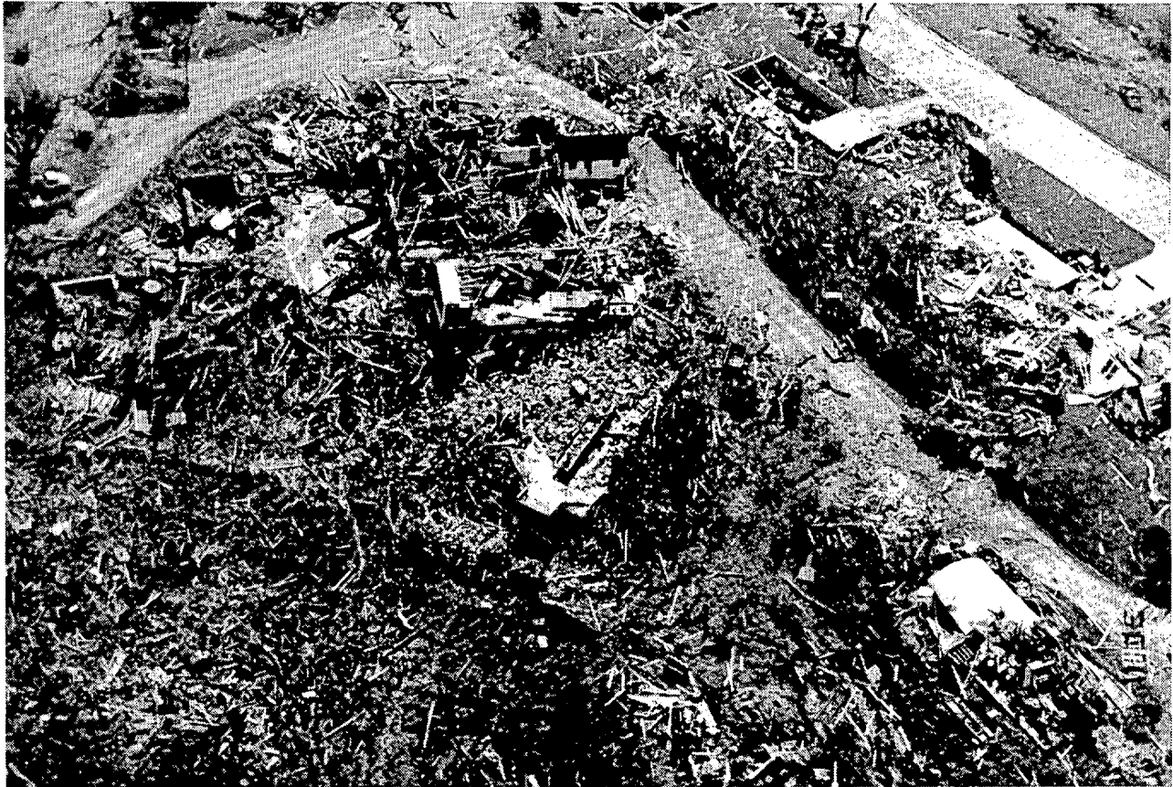
A destroyed farm on the southwest end of town, and nearby foundations where homes once stood. (CT)
