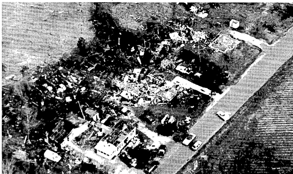
F2 (lower left) to F4 (upper right) damage done by the Bennettville Tornado along a street at Lester, SC.
