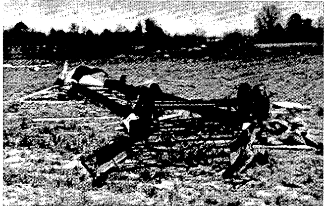
A bent mobile home frame after having been tossed about by the Mount Olive Tornado.
