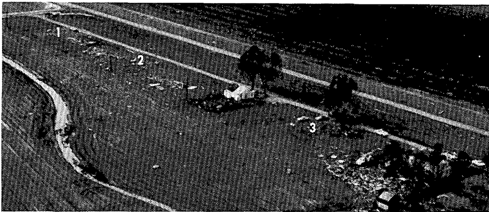
Three sites of destroyed homes where injuries occurred at the beginning of the damage path (looking northwest).
