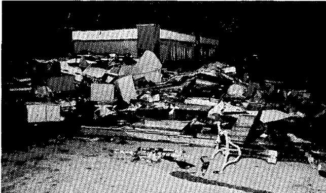
Band instruments and debris strewn from the destroyed building. Total damage to the school was estimated at $500,000.
