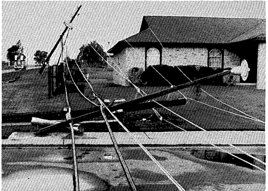
LEFT: A power pole remains standing after having been snapped off and moved several feet away by the microburst winds. ---Photo by Jim Wolfe, The Tulsa World. RIGHT: One of 10 power poles that were toppled across the road from the high school. ---Photo by Dick Grant, The Tulsa Tribune.
