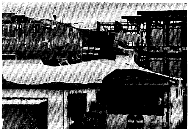
Roof damage to homes in Hawthorne.
