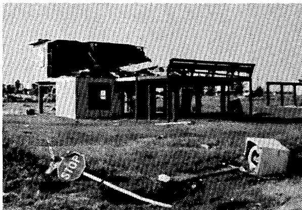
Wind-destroyed homes at Jamaica Beach, about 11 miles southwest of Galveston. Note that in the right photo, one home was blown apart while an adjacent home of the same design and construction appears untouched.
