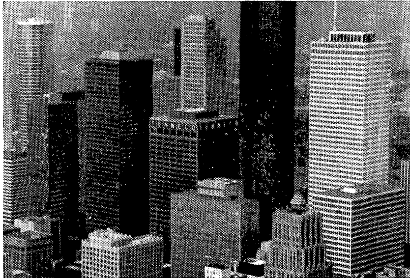
The skyscrapers of Downtown Houston with numerous windows boarded up. It is likely that the majority of the broken panes were caused by the impact of flying debris.
