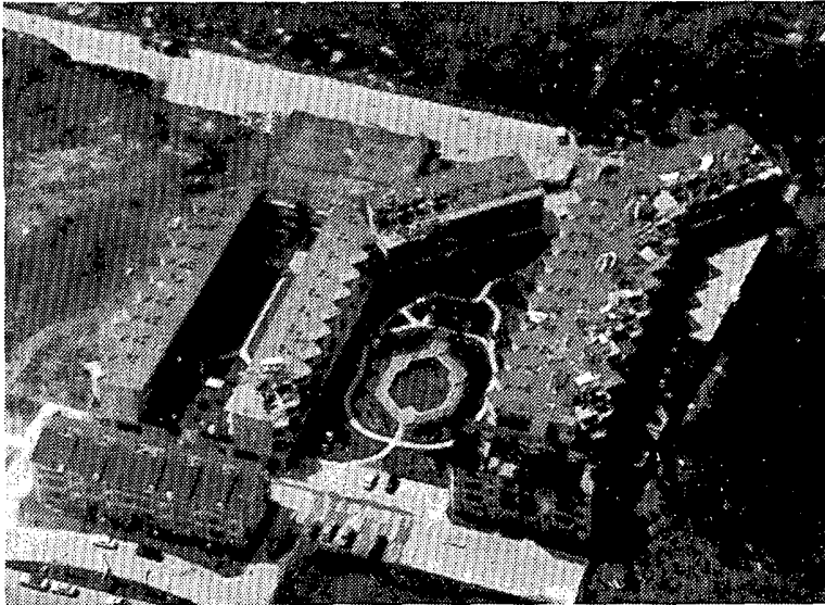
LEFT: Roofing torn from a hotel in Galveston.
