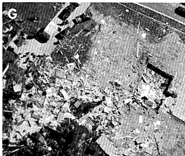
Samples of damage from the Andover, Minnesota Tornado. In photo (F), the homes on one side of the street lost their roofs while similar homes on the opposite side were spared. The home in photo (G) depicts F4 damage (estimated winds of 207-260 mph).
